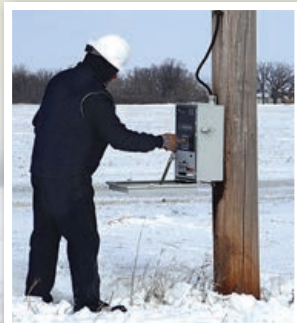
Thronson programs the regulator panel to maintain the voltage on the overhead power line.
