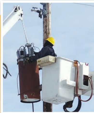
Cardinal, with help from Derosier operating the winch, removes the old regulator from the pole and lowers it to the ground. Derosier holds the new regulator in place with the winch while Cardinal lines the regulator up into position before he fastens it to the pole.
