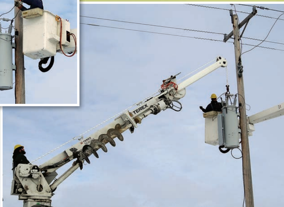
Journeyman lineman Aaron Derosier (operating winch) places the regulator back in the "tub" with hand gesture guidance from journeyman lineman Darcy Cardinal.
