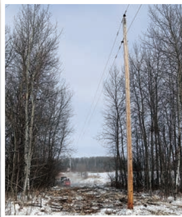
A before and after picture of some small brush that was hydro-axed using the Bobcat and brush-hog attachment.
