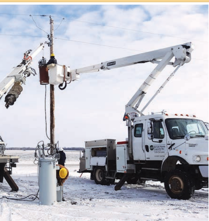
Cardinal, with help from Derosier operating the winch, removes the old regulator from the pole and lowers it to the ground. Derosier holds the new regulator in place with the winch while Cardinal lines the regulator up into position before he fastens it to the pole.
