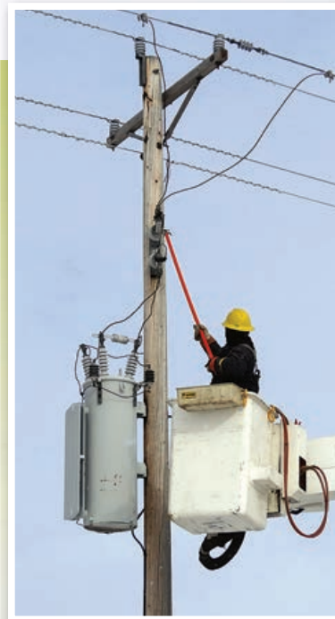
Journeyman lineman Darcy Cardinal uses a hot stick to take the regulator out of service to replace a faulted capacitor.
