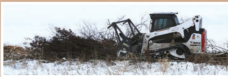
Journeyman lineman Jordon Gervais uses a “brush-hog” rotary brushing attachment powered by the Bobcat to clear vegetation in the power line right of way.
