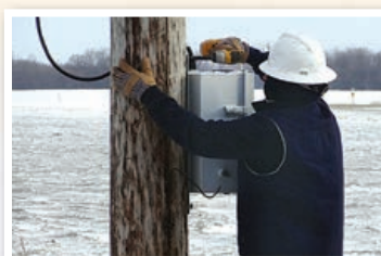
Cardinal, with help from Derosier operating the winch, removes the old regulator from the pole and lowers it to the ground. Derosier holds the new regulator in place with the winch while Cardinal lines the regulator up into position before he fastens it to the pole.
