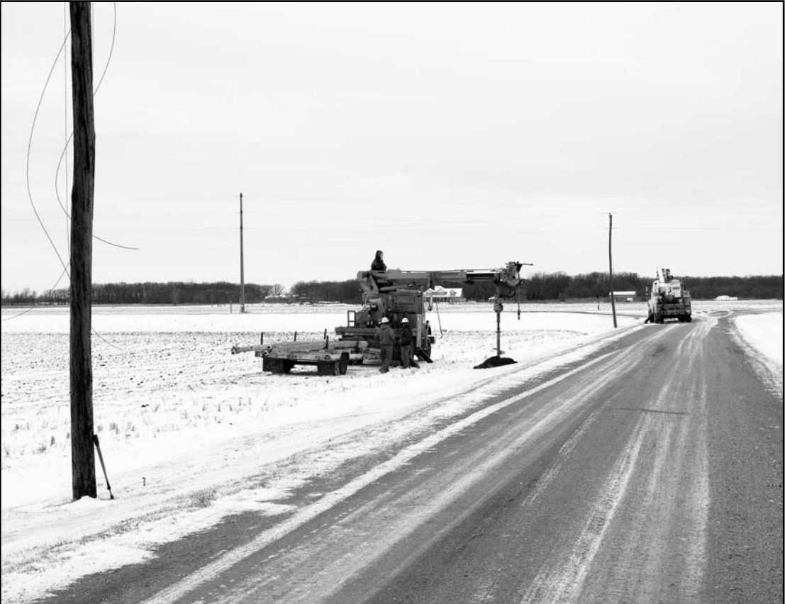
As the Red Lake Electric line crew works to replace the armeductor with ACSR, it requires an additional pole along the Hanson driveway. The ACSR can not be strung in the long spans that the armeductor could.
