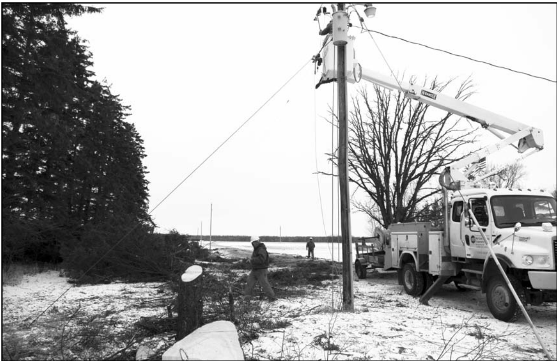
Red Lake Electric line personnel have the new ACSR wire strung and into place and work to restore electrical service into the Hanson farmyard. The Hanson farmstead did remain powered during the line conversion with the aid of their generator.
