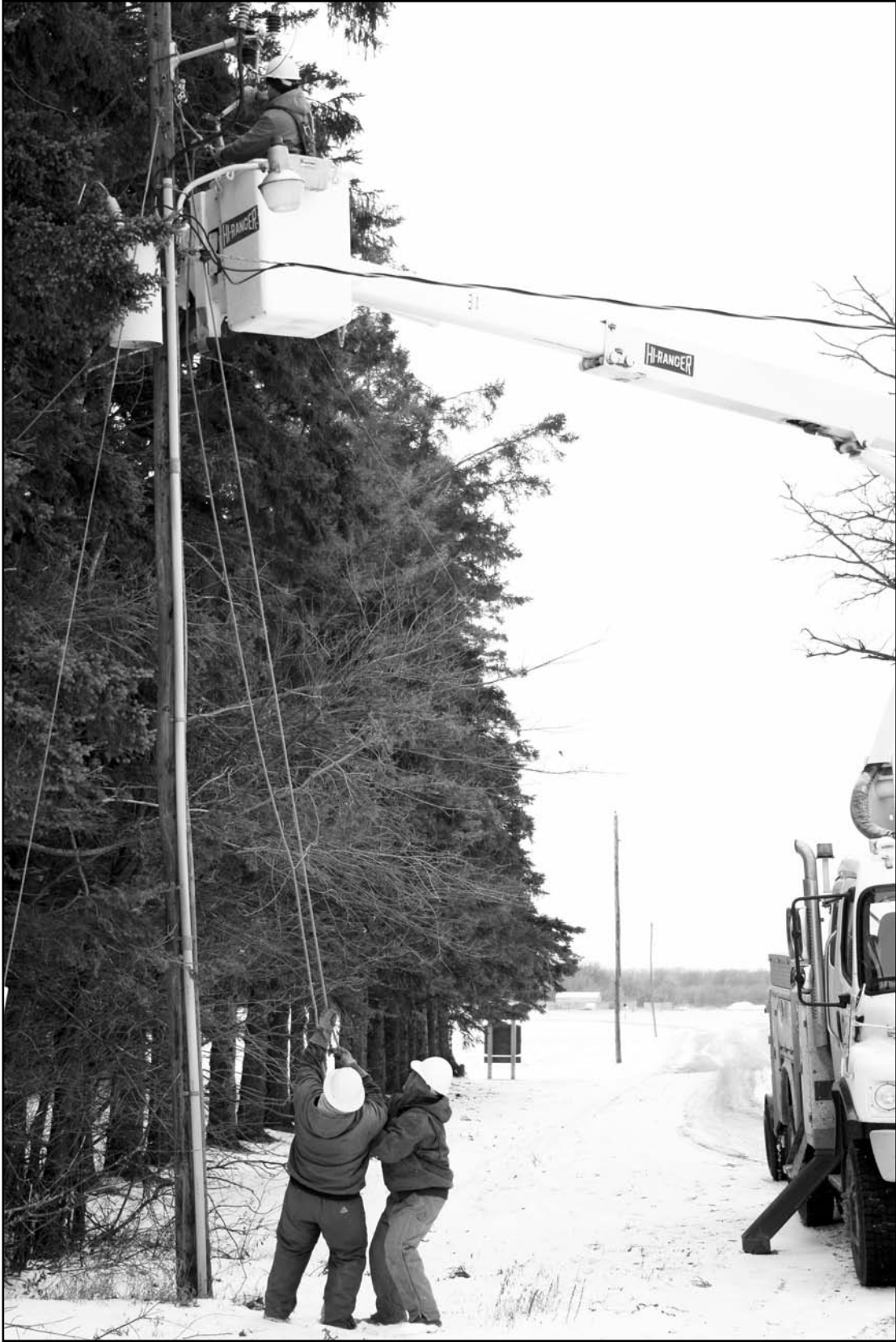
Red Lake Electric line personnel begin the task of replacing the armeductor wire into the yard of Wallace and Arlene Hanson of Viking. The linemen are dropping the conductor.
