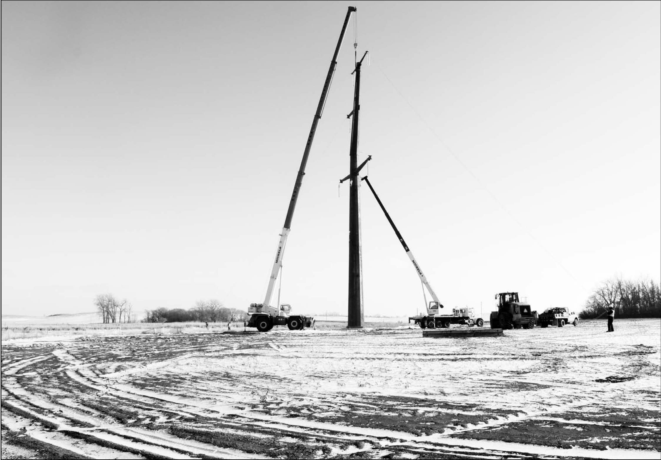
A structure is set in place for the center to Grand Forks transmission line that will stretch 250 miles across North Dakota.
