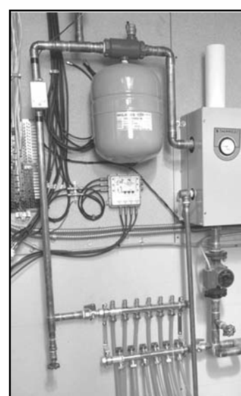
Electric Boiler-Slab Storage
