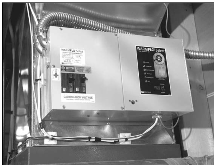
Electric Plenum Heater
