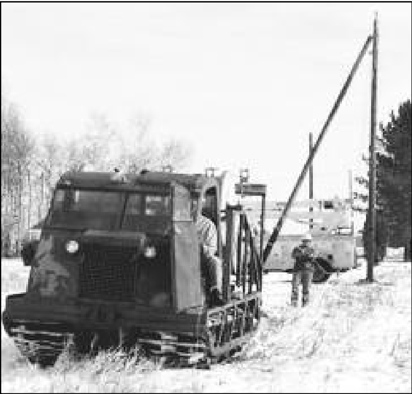
A Red Lake Electric line construction crew string wire for the line rebuild. The size of the new wire is 1/0 and the old wire was #4.
