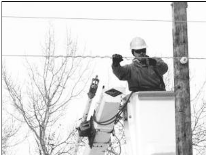
Troy Schmitz installs vibration dampeners on the new wires that have been strung for the line rebuild. The dampeners help prevent vibration from the wind to help keep the wire from fraying or breaking and to help keep the wire ties tight.
