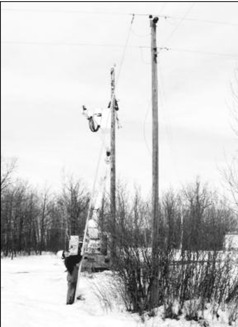
Casey Thronson uses an extendo stick to remove the hot tap for a service on an existing pole. The service tap will be moved to the new pole in the background.
