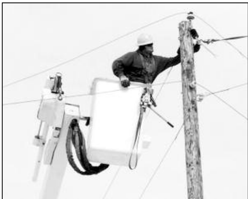
Travis Huot works to attach existing service wires to a new line pole that has been installed along Marshall County Road 30.
