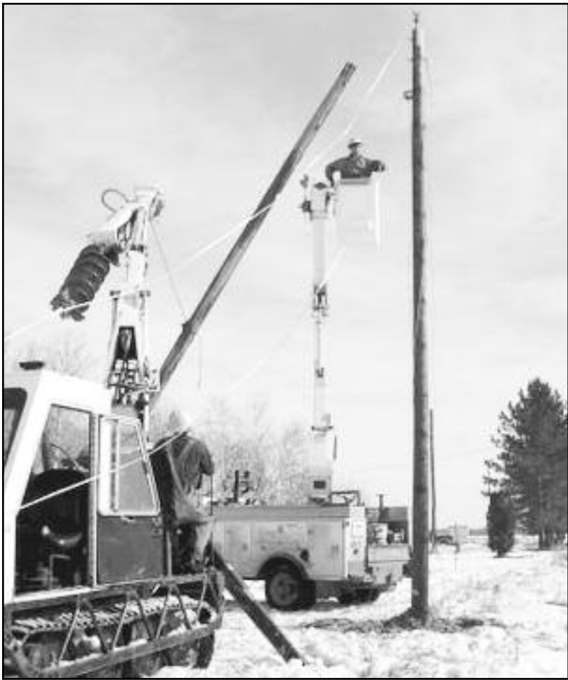
Red Lake Electric line workers are installing a push brace on an angle pole along county road 30. Once the road work is done an anchor and guy wire will be installed and the push brace will be removed.
