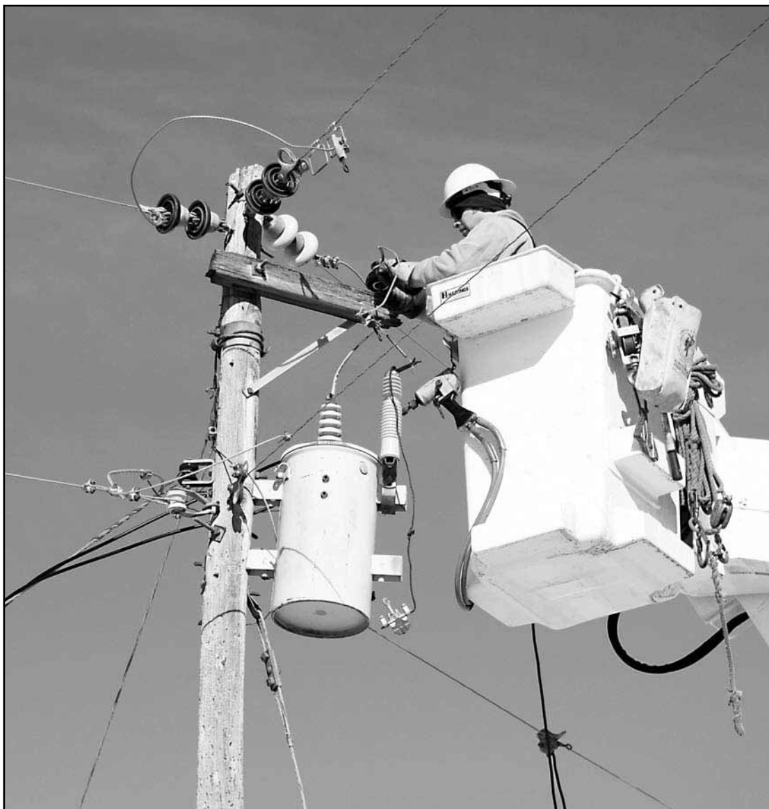
The change out of this rotten pole begins with Casey Thronson removing all of the hardware. The triplex going from this transformer pole to a meter pole will be changed to primary wire and the transformer will be moved to the meter pole.
