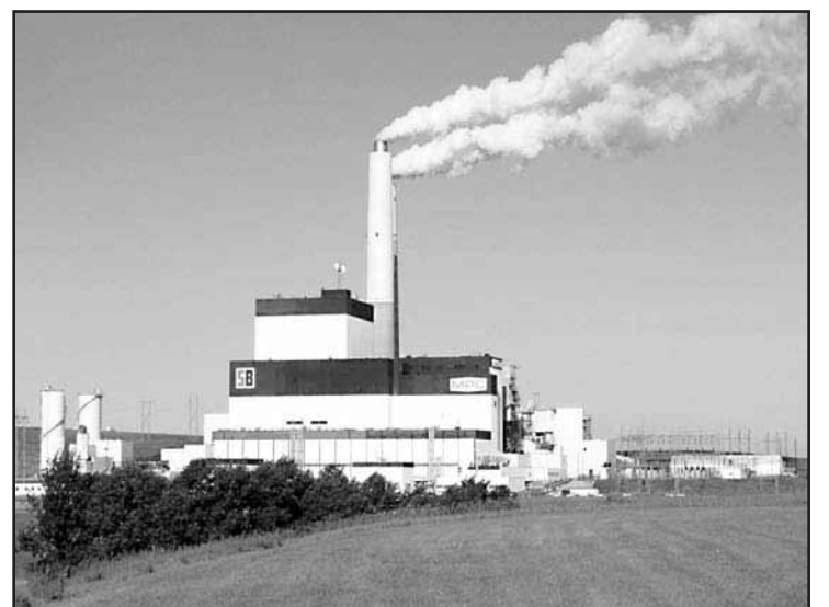
Minnkota Power Cooperative, Grand Forks, ND is using clean coal technology at the Milton R. Young Station near Center, ND. It was the first lignite-based, cyclone boiler power plant in the country to use CyClean Technology. CyClean reduces the emission levels of the power plant and helps provide a cost effective option to meeting future regulatory requirements.
