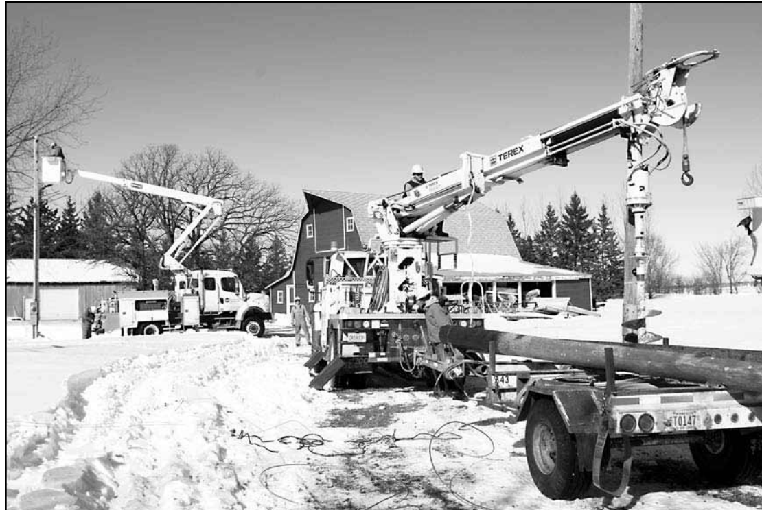
Red Lake Electric line personnel work in this yard south of Thief River Falls. The pole in the foreground is the rotten one being replaced. The pole in the background is where the transformer will be rehung. The work and maneuvering of trucks was made much easier thanks to the property owner who did the snow removal.
