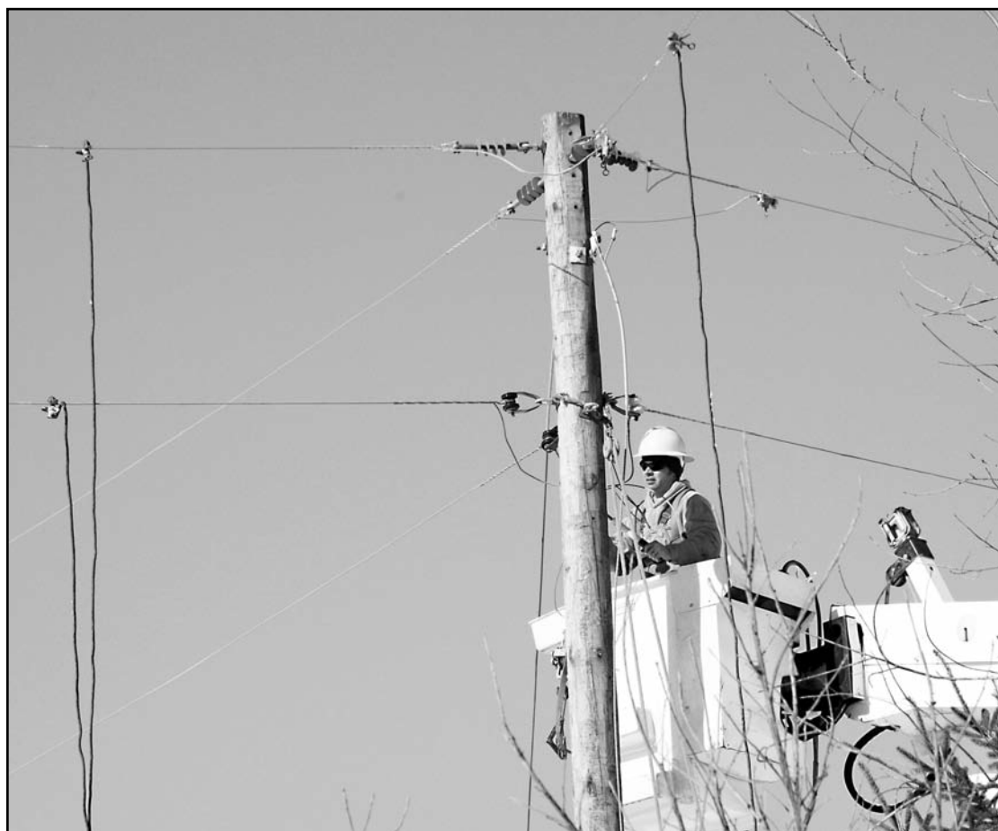
Casey Thronson works to attach all of the wires to the newly replaced pole. It is a 4-way dead-end pole with wires from four directions being attached to the pole. Wires from three of the directions could be possible power sources. Even though the line has been turned off, all three are grounded out with jumpers to provide added protection during the conversion process. The three hanging insulated wires are the ground jumpers.
