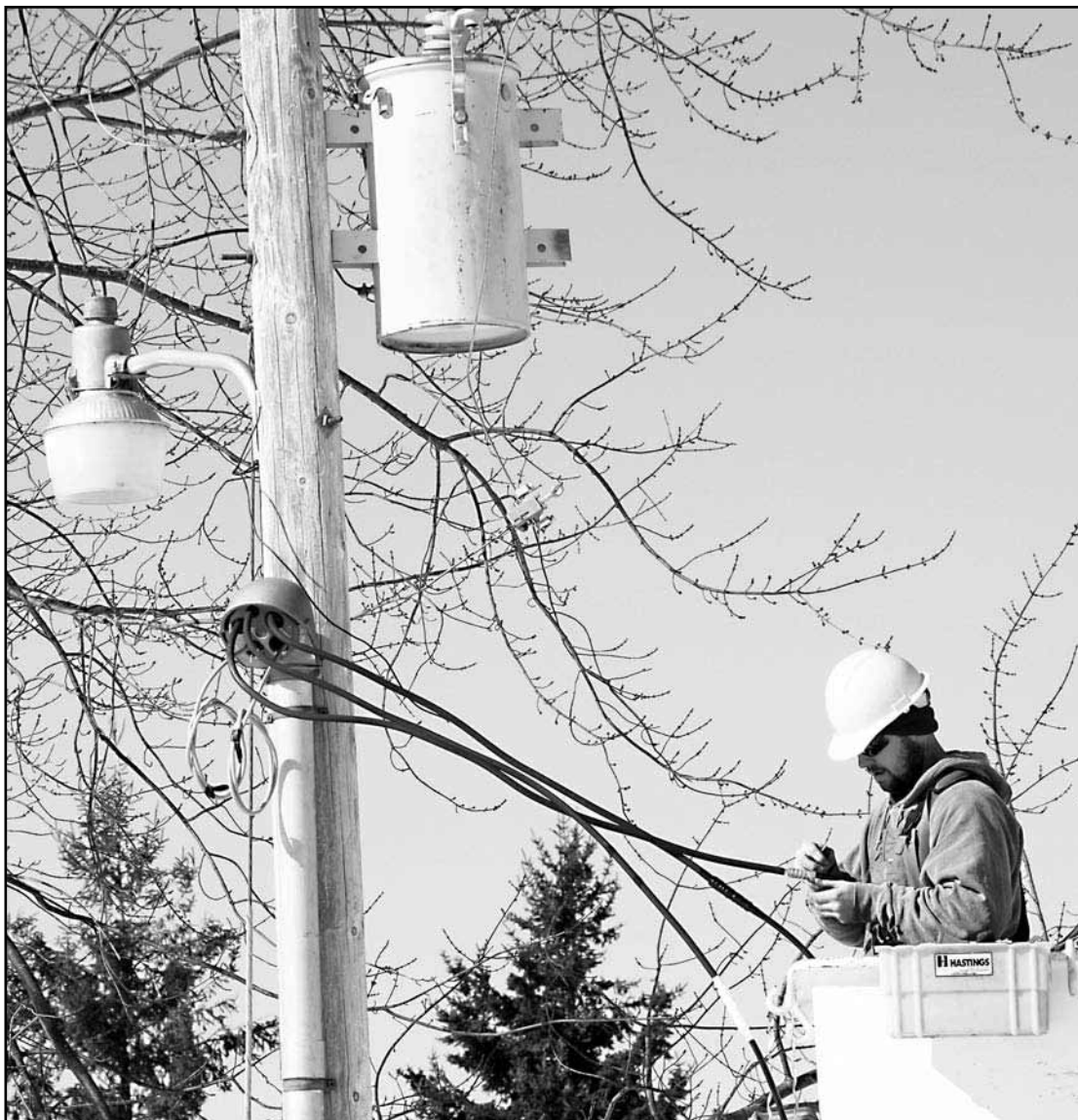
The transformer has been hung and Aaron Derosier works to splice extensions onto the tails of the wire for the meter loop so the wires can be connected to the transformer lugs.
