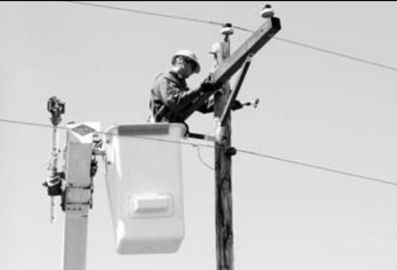
Brett Knott, apprentice lineman, attaches a crossarm to an existing single-phase pole. The poles along County Road 13 in Parnell Township were all replaced four years ago and are of sufficient height to accomodate a three-phase line.
