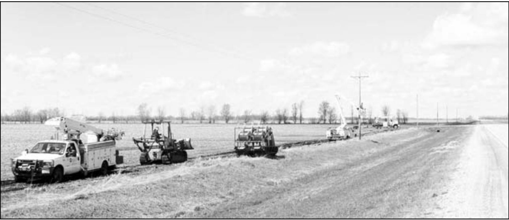
Above: A Red Lake Electric construction crew strings wire for the three-phase line upgrade along County Road 13 northeast of Crookston. A track dozer was used to pull trucks through the wet fields.
