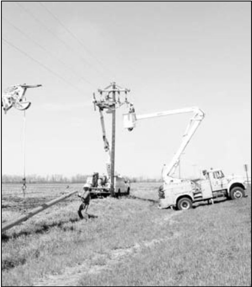
A line construction crew works on a new three-phase breaker pole and de-frames the old single-phase pole.
