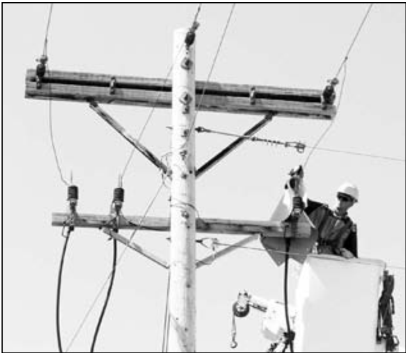
Brett Knott places an insulated blanket over a lightning arrester and epoxilator as he prepares to work on the three-phase pole. Covering this phase helps protect him from different potentials as he will be working on one of the other phases.
