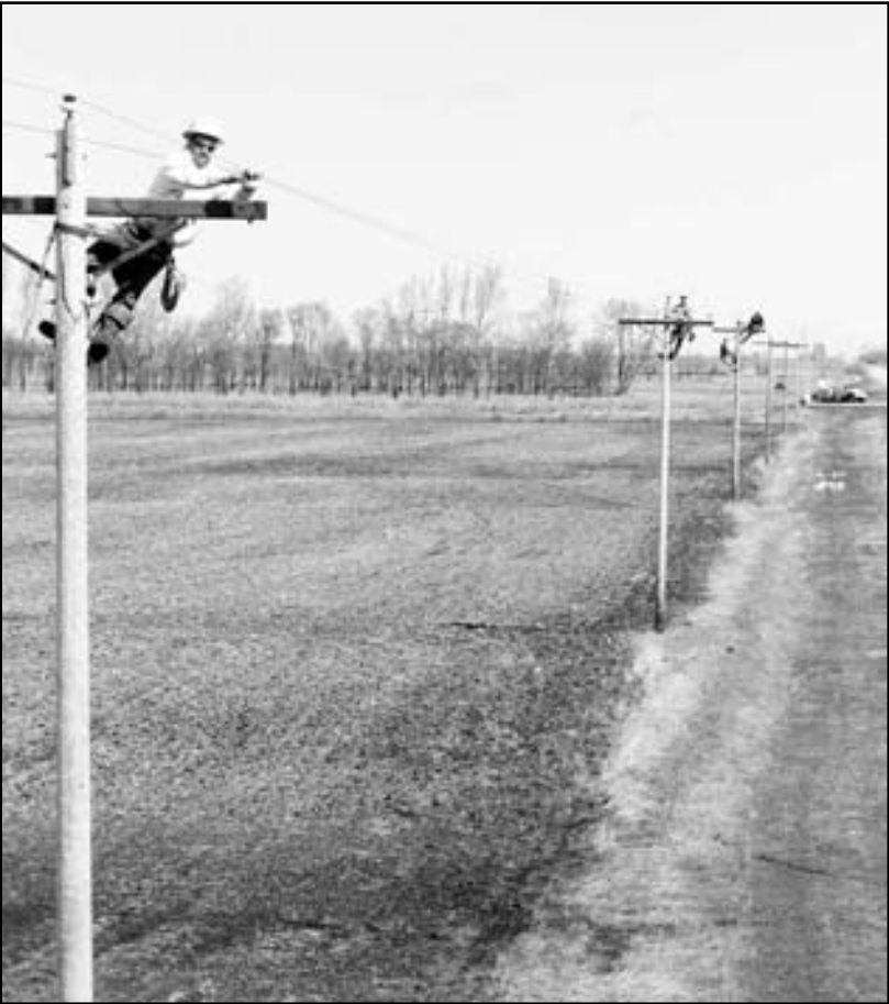
Above: A Red Lake Electric construction crew strings wire for the three-phase line upgrade along County Road 13 northeast of Crookston. A track dozer was used to pull trucks through the wet fields.
