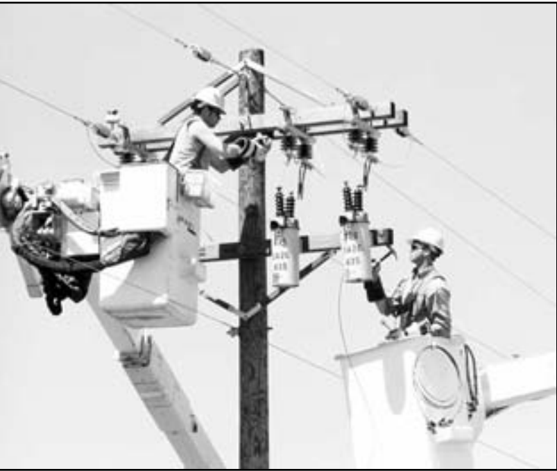
Casey Thronson, left, lineman, and Brett Knott work to complete the attachments on the three-phase breaker pole. A breaker isolates a section of line so if a fault occurs down-line it will open the breaker allowing electric service to remain for services up-line.
