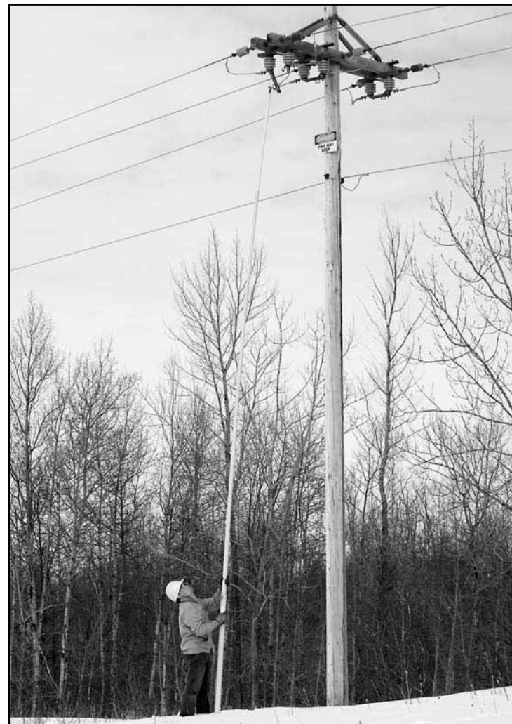
This is one of several two-way feed poles that were closed during the Dakota substation outage in order to minimize the number of accounts to be without electrical service. Red Lake Electric apprentice lineman Aaron Derosier uses an extendo stick to open the feeds once the substation was re-energized.
