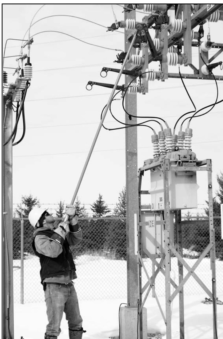
Red Lake Electric lineman, Brett Knott uses a fiberglass stick to open every blade on every breaker in the Dakota substation when the substation was taken out of service. There are five circuits each with a three phase breaker requiring 15 blades to be opened.
