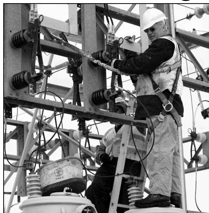
Once the substation was de-energized and everything ground out, Minnkota Power Cooperative line personnel changed out the broken insulator.
