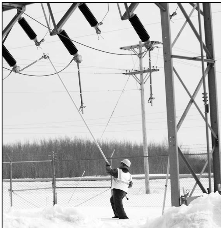
Red Lake Electric lineman, Brett Knott uses a fiberglass stick to open every blade on every breaker in the Dakota substation when the substation was taken out of service. There are five circuits each with a three phase breaker requiring 15 blades to be opened.
