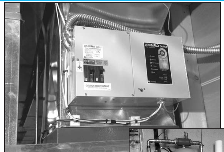
Electric Plenum Heater (Above)
