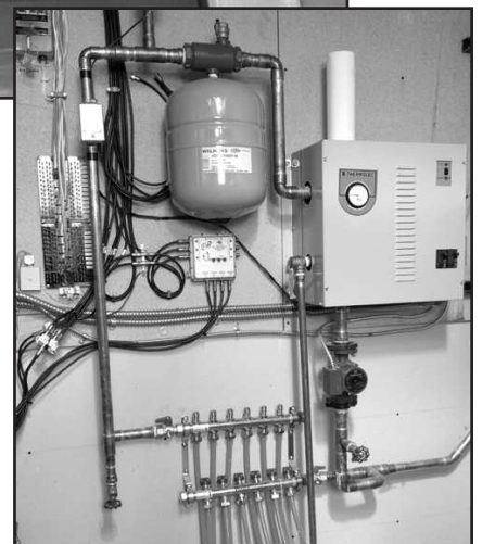
Electric Boiler-Slab Storage (Right)
