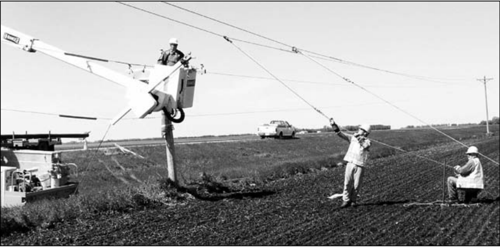
Two phase wires are tied-off and held out of the way, with link sticks, as part of the preparation to change out the pole.
