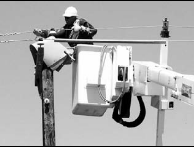
The replacement pole is in place and Alan Cota ties-in the wires onto the insulators. Rubber blankets and sleeves are used to cover-up items of different potential from the wire he is working on. The process of changing out the pole takes place with each phase wire energized with 7,200 volts. There was no disruption of electrical service to any member during the change out. Another pole replaced, hopefully to serve 40 to 50 years or more.
