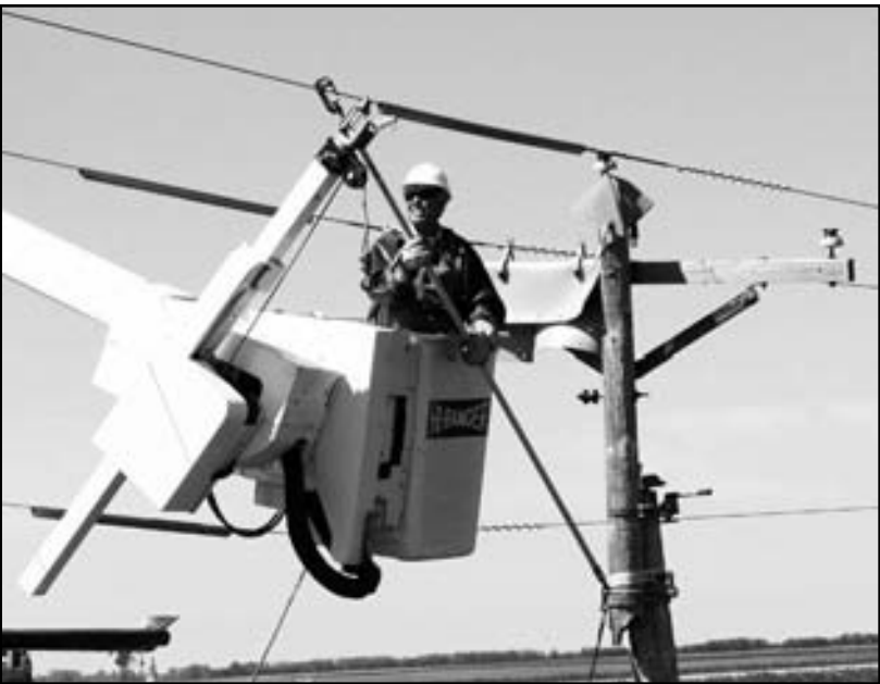
Right: Alan Cota, linecrew foreman, attaches a link stick to a phase wire as he prepares to un-tie all the wires on the damaged pole.
