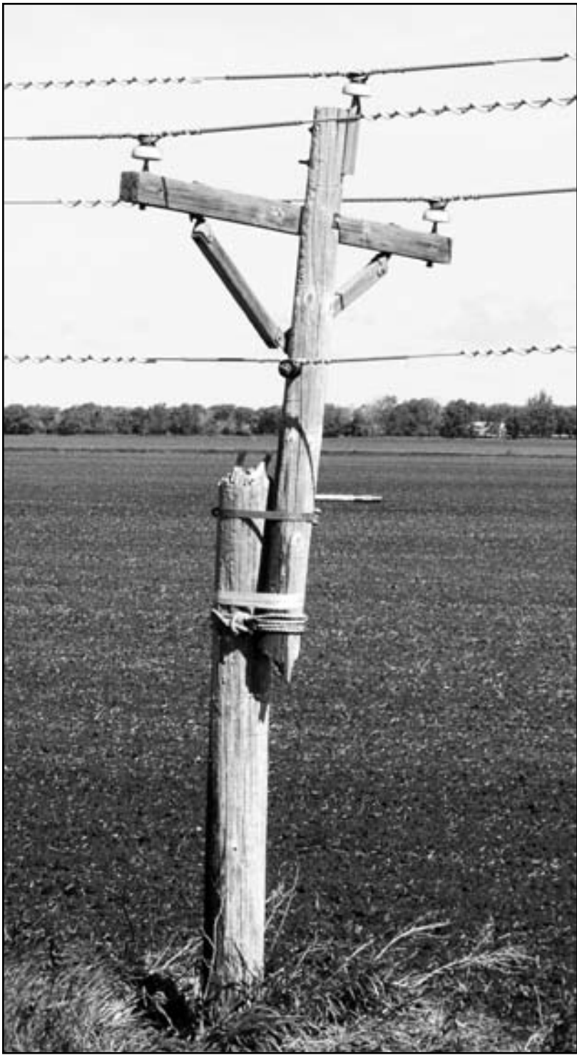
This three-phase pole was broken by strong winds. During restoration work the upper part of the pole was secured to the pole butt until the pole could be replaced at a later time.
