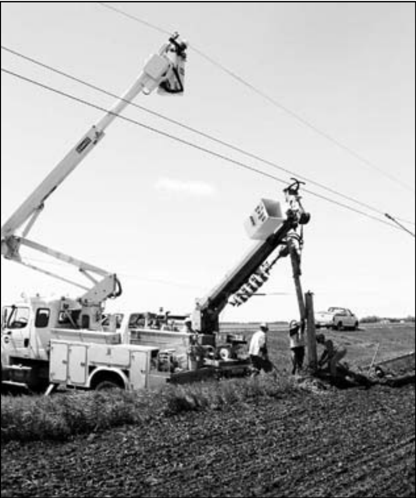
The third phase wire is held up and out of the way in the jib of the bucket truck. The neutral wire has been tied off to the rear hitch of the truck. With all of the wires out of the way, the pole can be changed out. The work is done from the ditch side in order to prevent driving on the seeded field.
