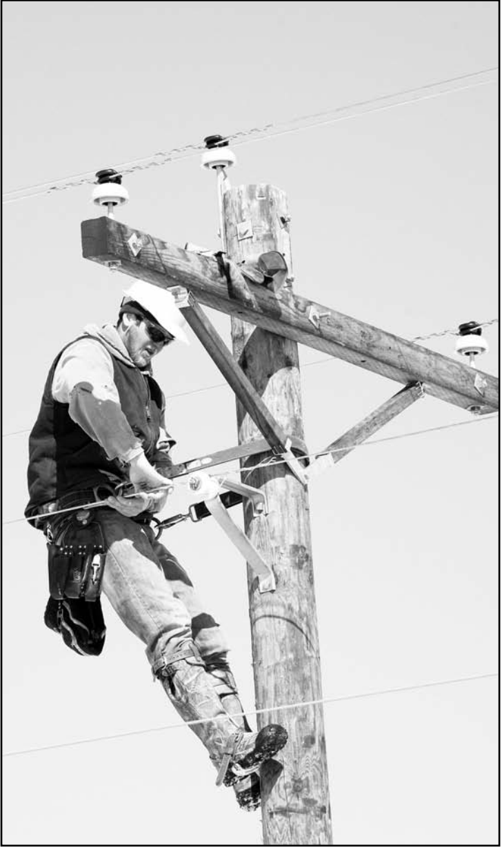
Brett Knott, lineman, uses preformed ties to attach the wires to the insulators of the new three phase line.
