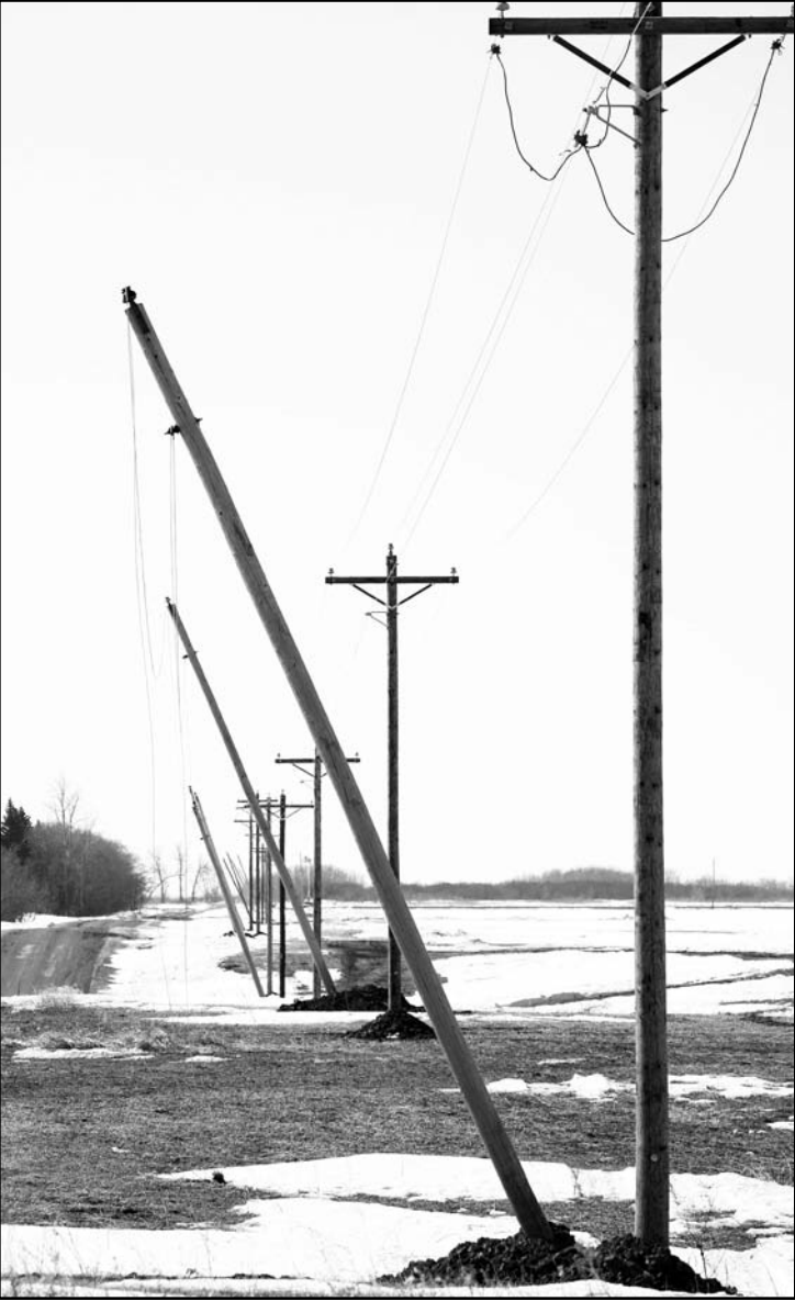
Red Lake Electric line crew personnel set the old single phase poles at an angle so the new three phase poles could be set in line
