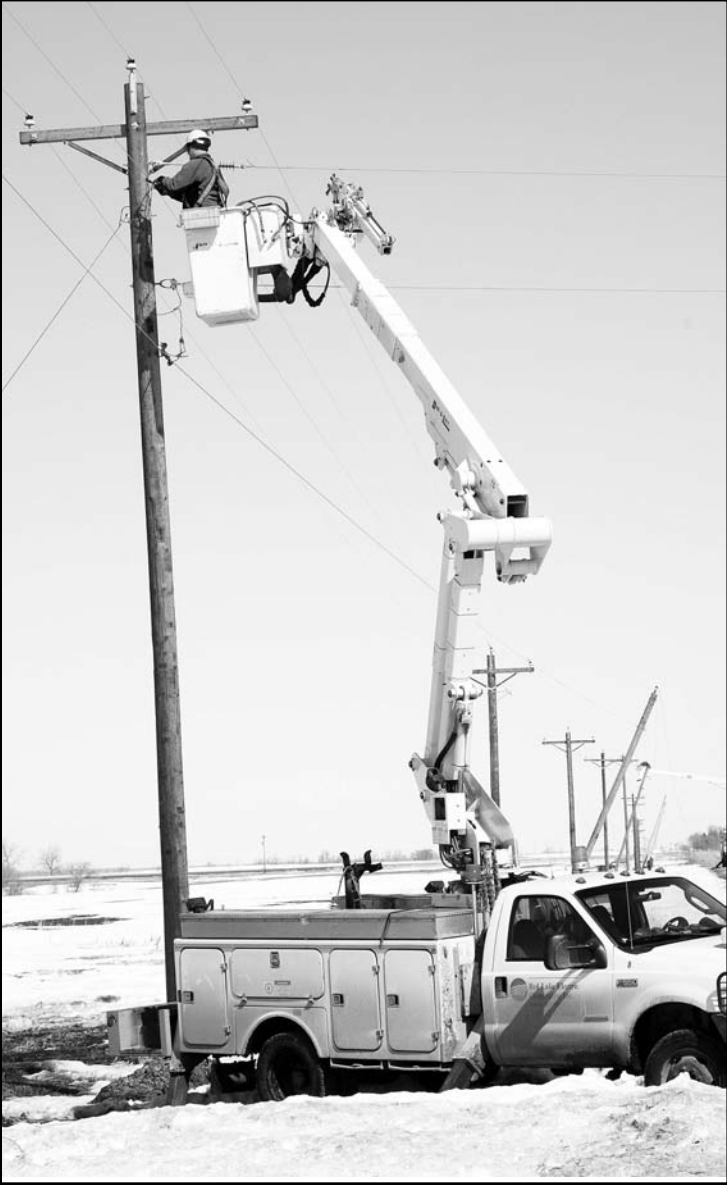
Cooperative crews work to put the finishing touches on the new three phase line.
