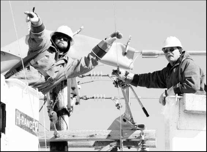
Sam Pahlen (left) and Steve Kruse check the wires on the new three phase line for proper tension and sag.
