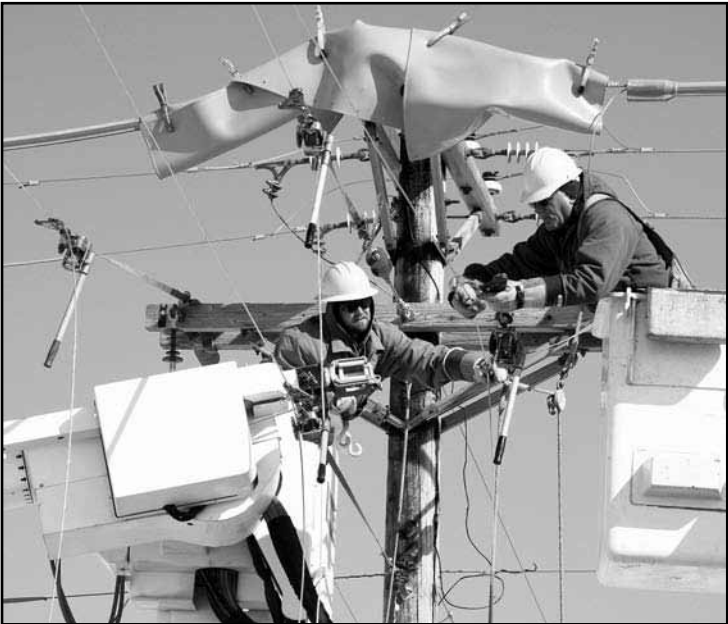
Sam Pahlen (left), apprentice lineman and Steve Kruse, lead lineman work to attach the wires for the new three phase line to an existing three phase take-off pole.
