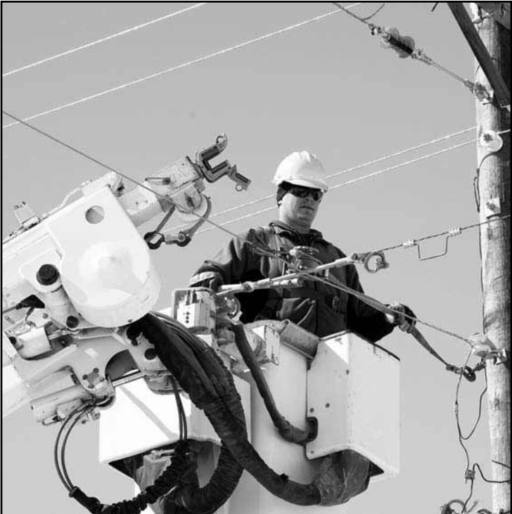
Jordan Gervais, apprentice lineman, works to reconnect a single phase tap into an existing farm yard, onto a new pole.
