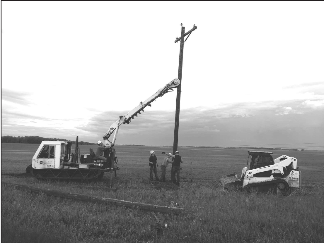
Red Lake Electric line crews use a track digger to set a new pole northwest of Red Lake Falls. The old pole was broke as a result of strong winds on May 28.
