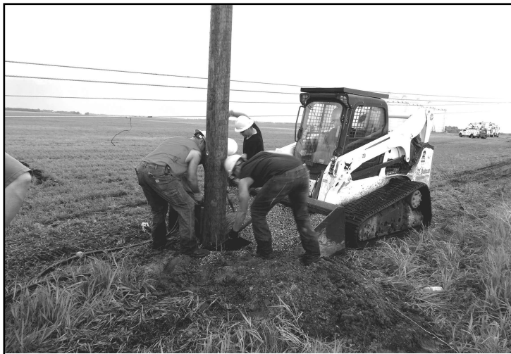
(Above) Red Lake Electric line crews set a new pole northwest of Red Lake Falls. The old pole was broke as a result of strong winds on May 28.
