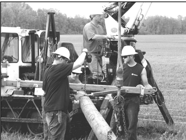
Red Lake Electric linemen Jordon Gervais (left), Brandon Narlock (center) and Brett Knott (right) work together as they frame a new three-phase pole. Crew foreman Troy Schmitz (back) operates the track digger as he drills a hole to set the new pole.
