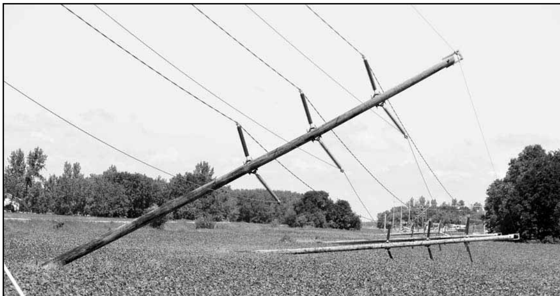
One mile of transmission line poles were toppled by the strong winds of the micro burst that traveled through the area east of Thief River Falls on July 12. These poles are located south of Minnkota Power Cooperative's 115 KV substation located east of Thief River Falls along Highway 1.
