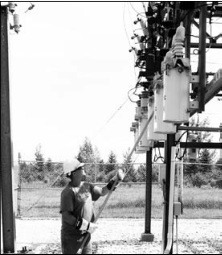
The substation had been bypassed and taken offline for the change out of the insulator. Red Lake Electric apprentice lineman Jordan Gervais uses an insulated fiberglass stick to open all of the breakers in the substation.
