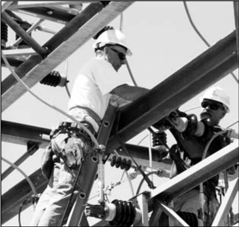
The substation had been bypassed and taken offline for the change out of the insulator. Red Lake Electric apprentice lineman Jordan Gervais uses an insulated fiberglass stick to open all of the breakers in the substation.
