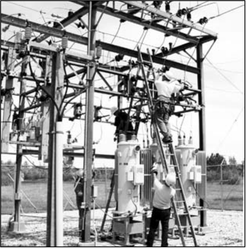
Minnkota Power line personnel and Red Lake Electric line personnel get set up and prepared to change out the burnt insulator.
