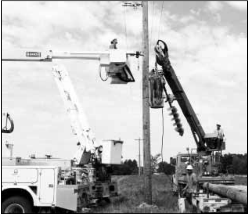
Lineworkers work to raise the regulator to be attached to the new three-phase pole. The connection process will begin as the regulator is cut-in-line to be placed back into service.
