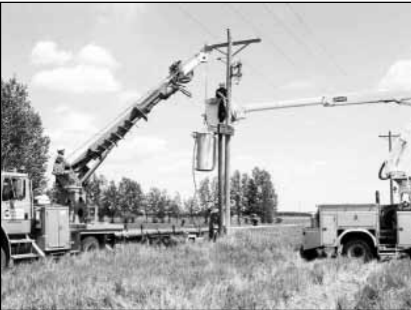
The regulator is lowered from the pole, which is to be removed, and will be remounted on the new pole.
