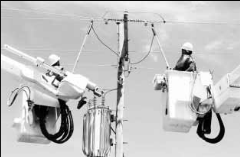
Red Lake Electric lineworker Sam Pahlen, left, and Troy Schmitz use shotgun sticks to simultaneously disconnect and remove the hot taps and leads that were connected to the regulator cutout.
