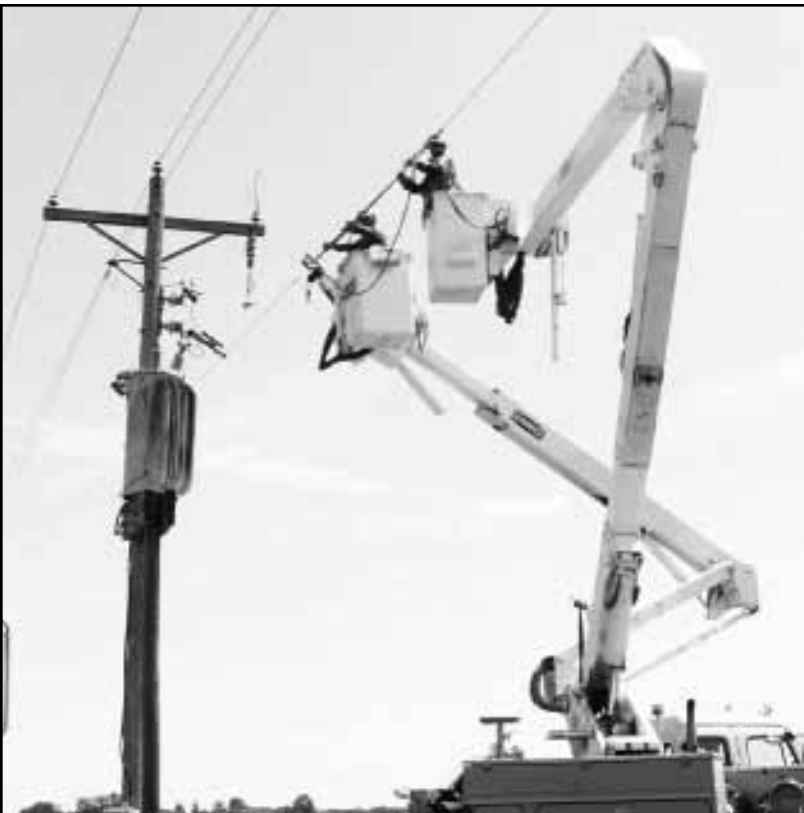
Schmitz and Pahlen work to remove the wires from the old three-phase regulator pole. With the wires now disconnected from the regulator, the wires leading to and from the regulator need to be connected; the crew accomplishes this by adding a splice to the wires.
