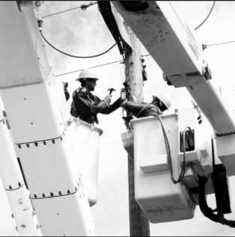
Pahlen, left, and Red Lake Electric lineworker Aaron Derosier work to mount the cutout for the regulator on the new pole.
