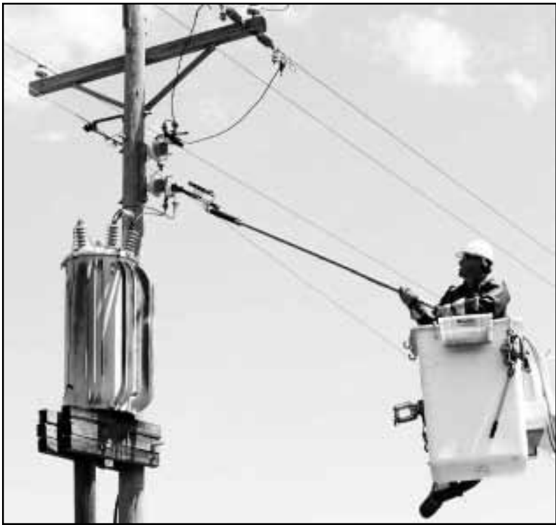
Red Lake Electric lineman Troy Schmitz uses a shotgun (insulated fiberglass) stick to open the cutout taking the regulator out of service.
