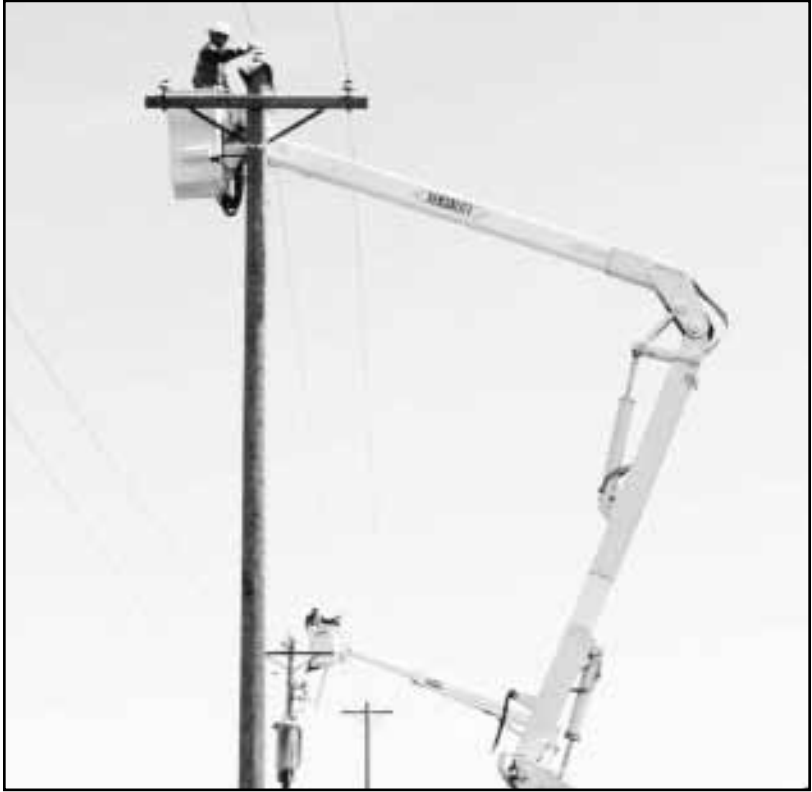
As all the wires have been disconnected from the old pole, Pahlen, in the foreground, begins to attach them to the insulators on the new regulator pole.
