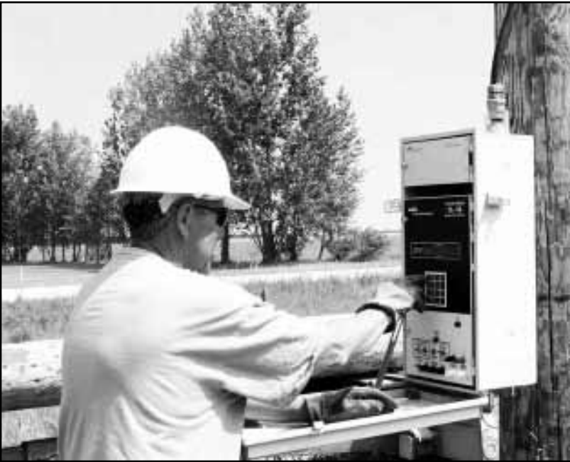
Once the regulator is reconnected, Alan Cota, crew foreman, checks the regulator control panel to make sure the regulator is operating properly. Another process completed in hopes of providing years of reliable service.
