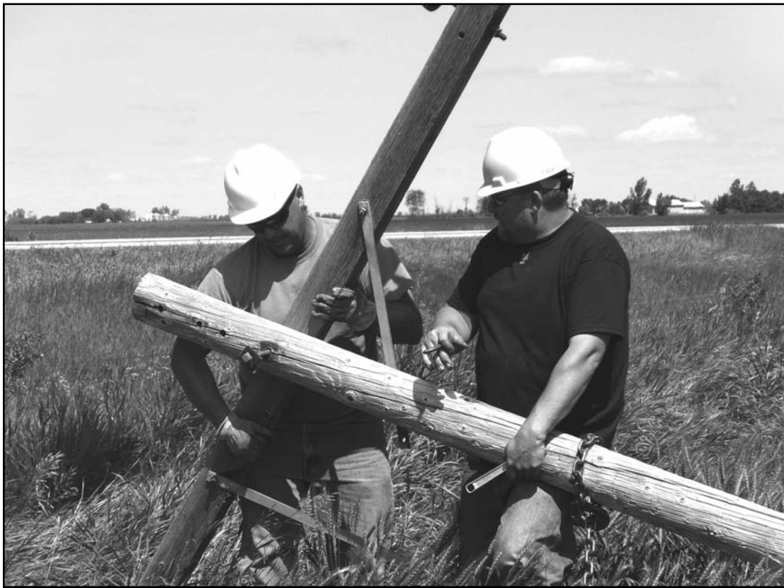
Red Lake Electric lineman Troy Schmitz (left) and PKM lineman Joe Marcotte (right) work together as they unframe a broken three-phase pole. Twenty five broken poles were reported as a result of the tornado that passed through the area on July 21.
