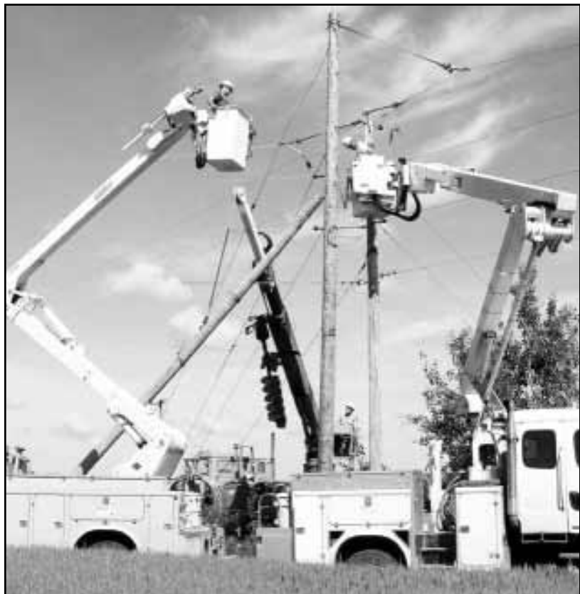
A Red Lake Electric line crew begins the transfer of material and wires from one three phase pole to another. The new pole had been set previously to help minimize the outage time.
