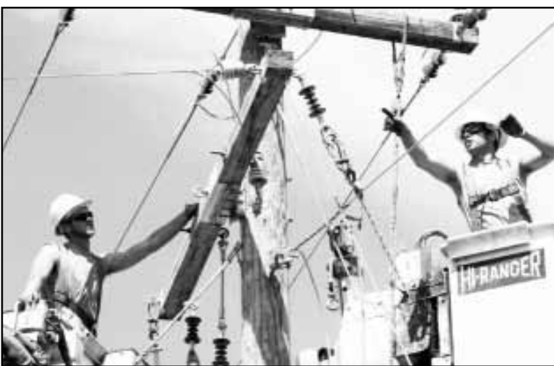
Brett Knott (L) and Casey Thronson (R) discuss which wires need to be connected together to complete the connections on the three phase pole.
