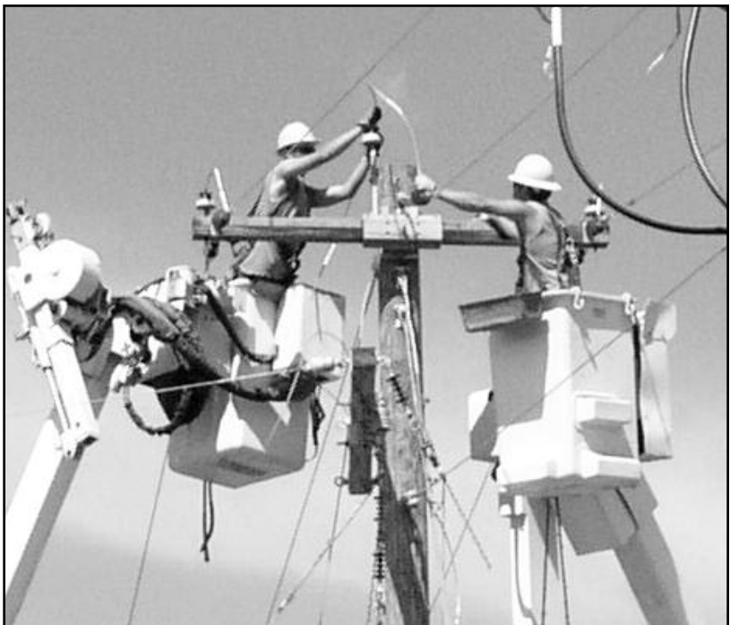
Another Red Lake Electric line crew works to attach material and wires to a three phase pole near the east end of the road upgrade. Wires on this pole are also connected to a new three phase underground riser pole that had been framed and set earlier.
