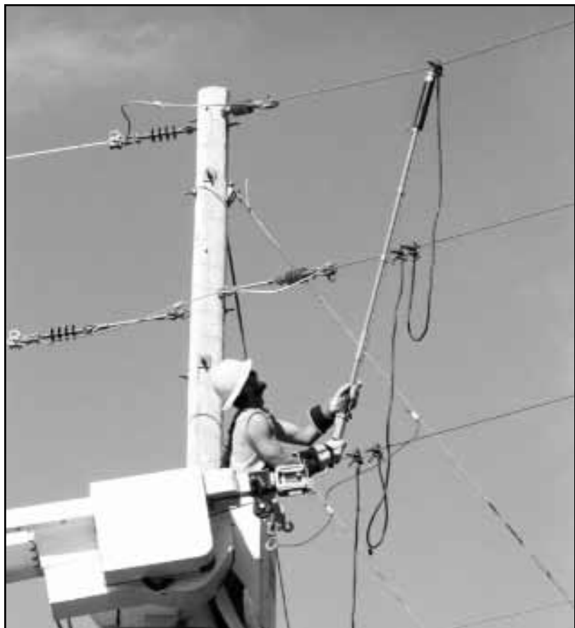
Sam Pahlen uses an insulated fiberglass shotgun stick to ground out all of the wires on a pole at the west end of County Road 31. All of the wires are connected together and grounded for the safety of those that will be working on the pole change outs.
