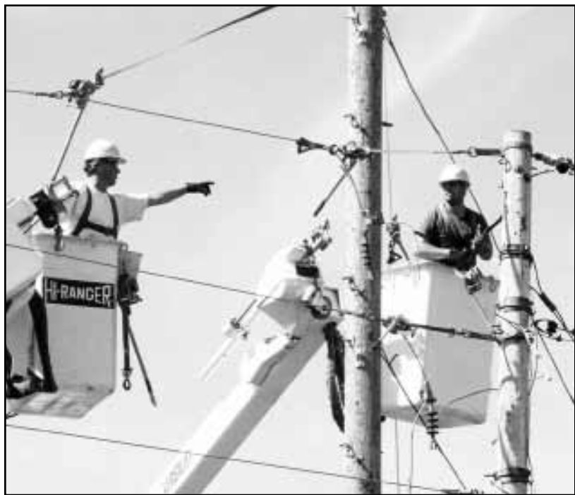
Troy Schmitz (L) and Aaron Derosier (R) use web hoists to loosen and remove the wires from the old three phase corner pole and to tighten and attach them to the new pole.
