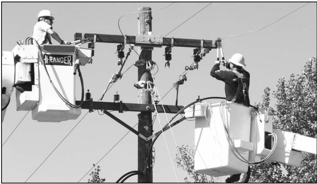
Red Lake Electric lineman Casey Thronson (left) and Branden Narlock cut the overhead wires prior to connecting the new underground cable.
