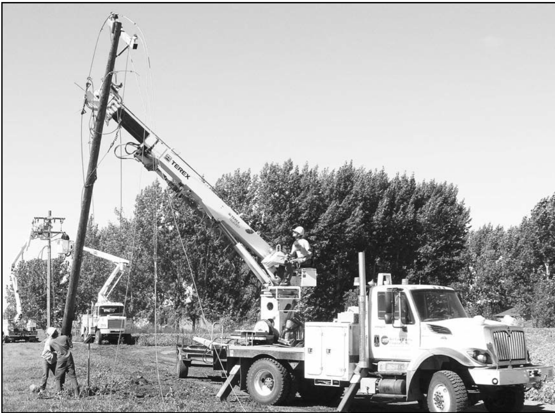
Five personnel work to remove and retire the overhead line that is being replaced with three spans of underground cable. The overhead line was replaced to allow for the ease of construction equipment to travel in and out of the contractors headquarters safely.
