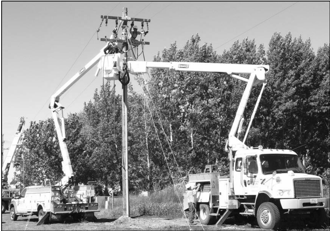
Red Lake Electric linemen begin the terminations on an underground riser pole where an existing overhead line is being replaced with an underground line.
