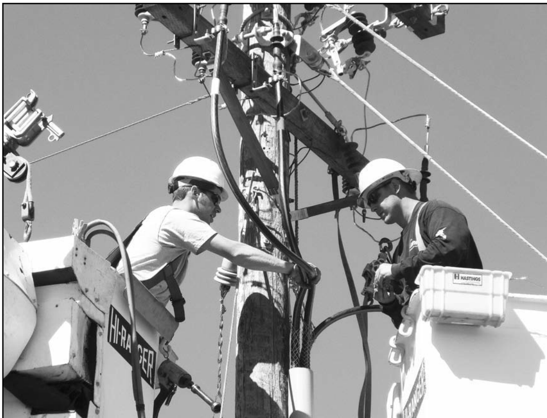
Thronson and Narlock make some of the final connections on the underground riser pole.
