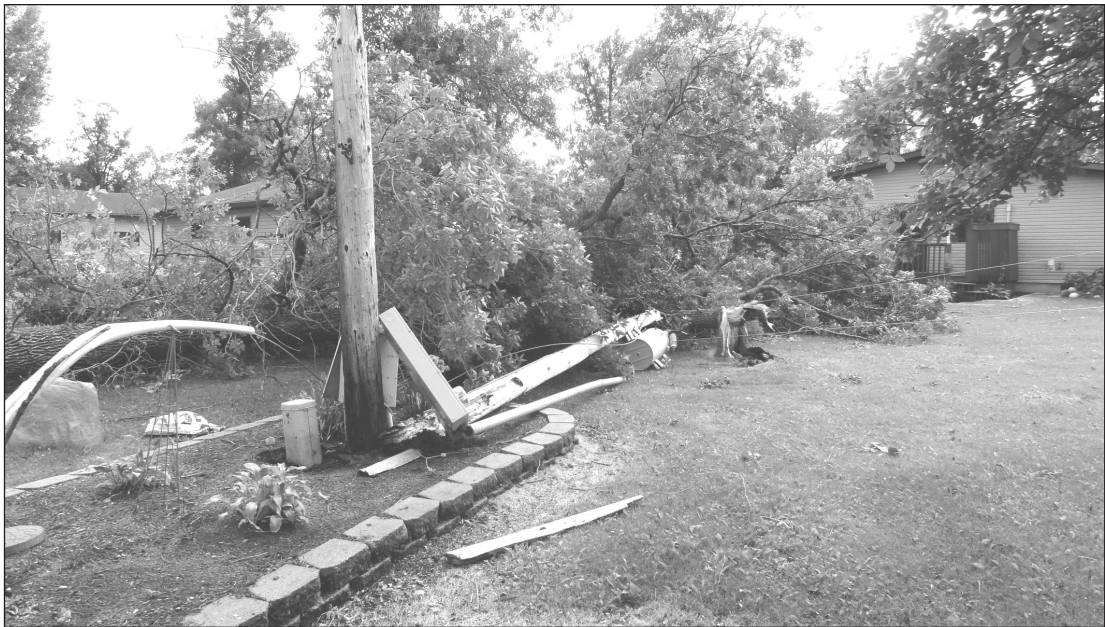
As a result of the excessive winds on August 12 a well-established tree fell into the overhead power lines breaking a Red Lake Electric pole.
