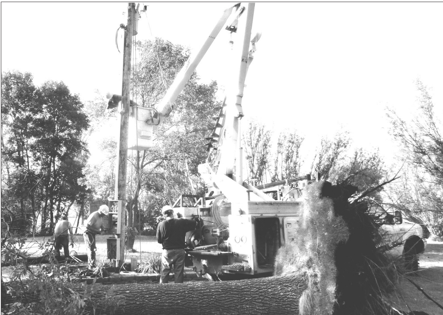
After a new pole was installed, RLEC crews work to connect new equipment on the pole that was needed to replace equipment damaged from the storm.
