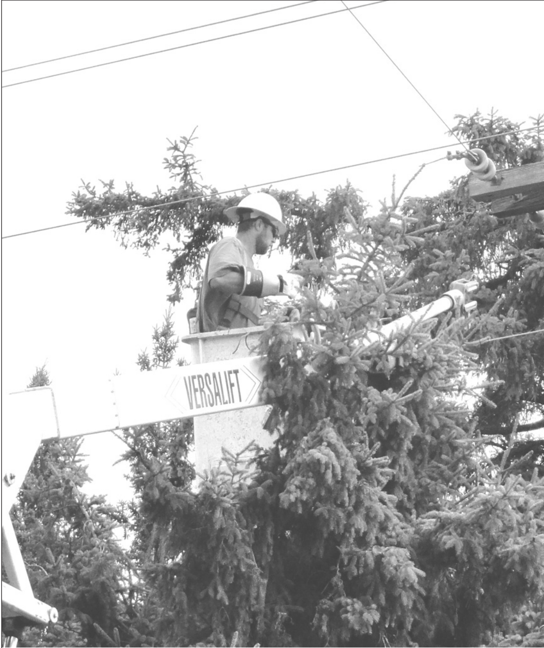
Red Lake Electric lineman Sam Pahlen trims an evergreen tree that has grown into Red Lake Electric's overhead power lines
