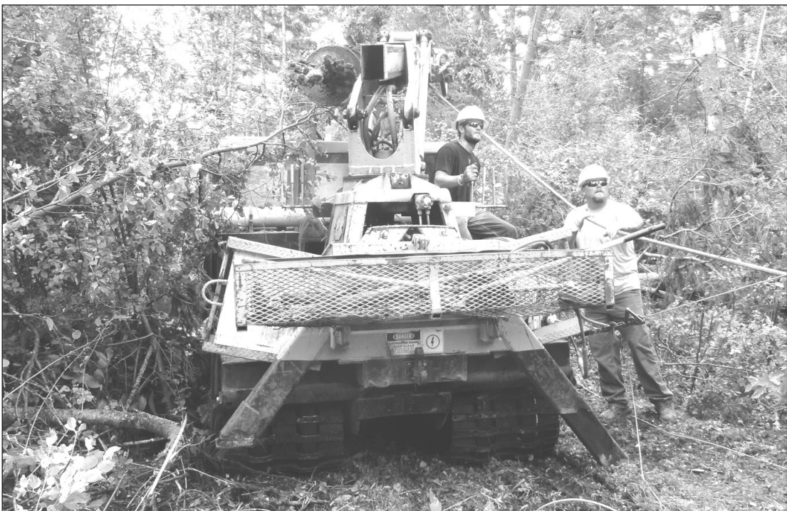
PKM lineman Nolan Knott (left) and Joe Marcotte (right) use a track digger to assist RLEC crews string a line which was taken down as a result of the straight line winds on Aug. 12.
