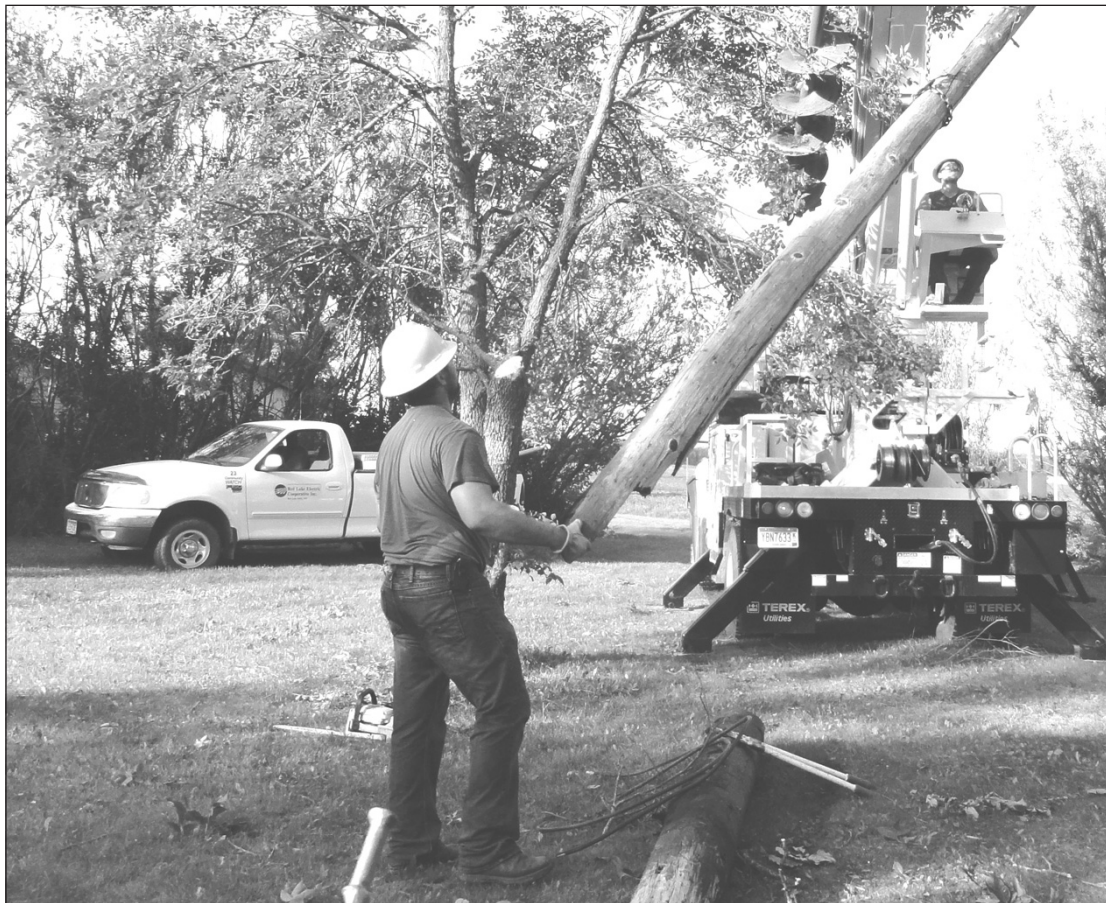
After a new pole was installed, RLEC crews work to connect new equipment on the pole that was needed to replace equipment damaged from the storm.
