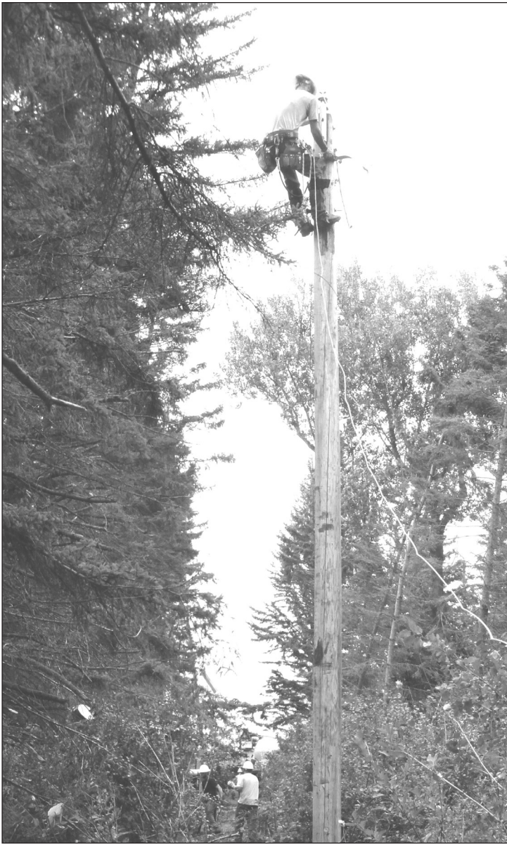
PKM lineman Ben Pahlen works to attach the overhead wires to the new pole that was installed.
