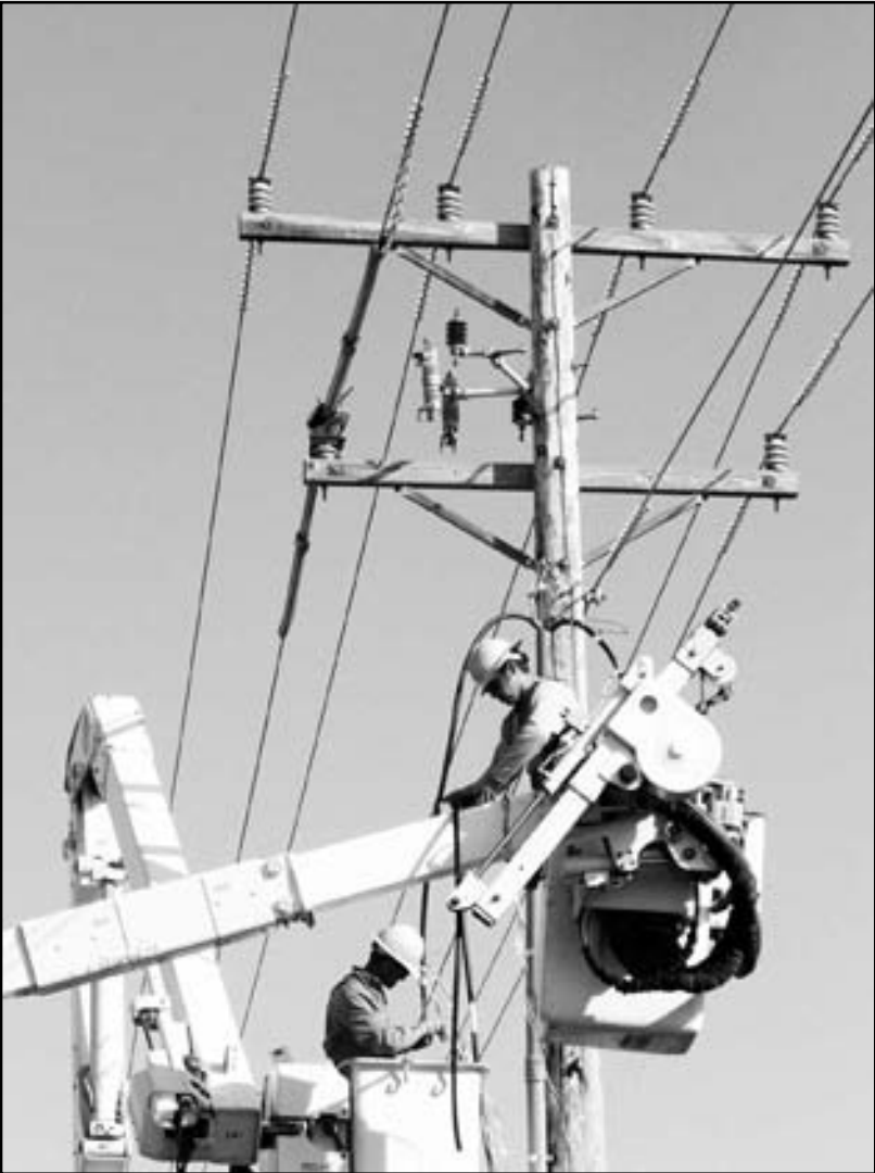
Brett Knott, in the lower bucket, and Casey Thronson work to prepare the ends of the underground wires prior to being attached to the terminator bracket. This new grain handling system required a 600 amp service.
