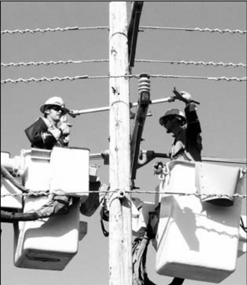
Casey Thronson, left, and Brett Knott work to attach a three phase terminator bracket to a three phase pole. The bracket will be used to hold the wire and other attachments for the new three phase service.
