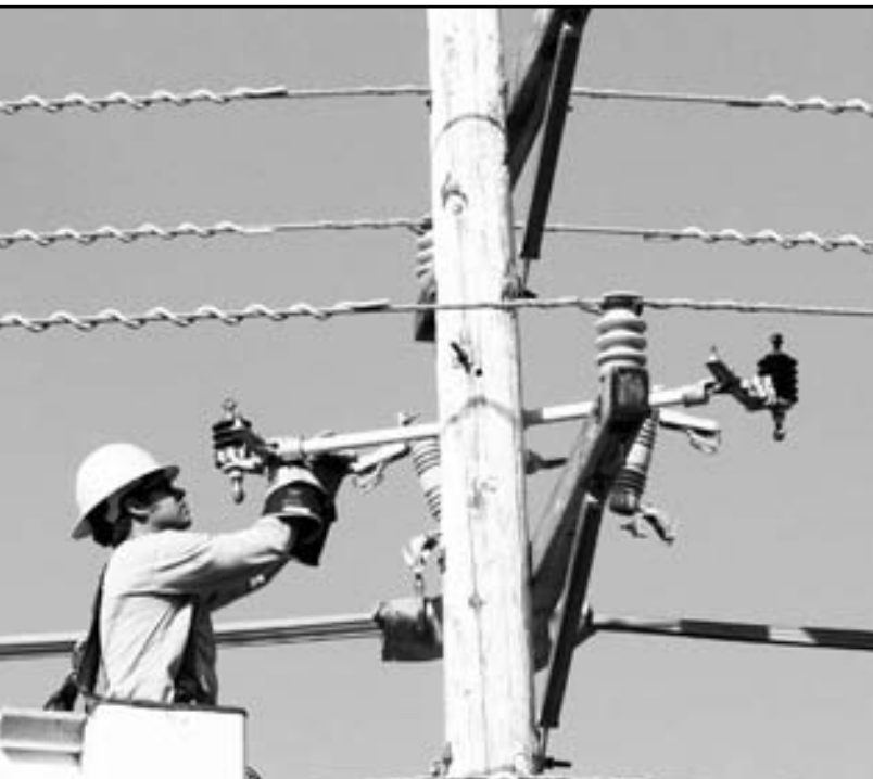
Casey Thronson installs lightning arrestors and fuse cutouts to the terminator bracket for the three underground wires. Lightning arrestors help protect the cable from lightning surges by bleeding off potential damaging charges to ground. Fuse cutouts are installed so the underground service can be disconnected or opened without interruption to the overhead feeder line.
