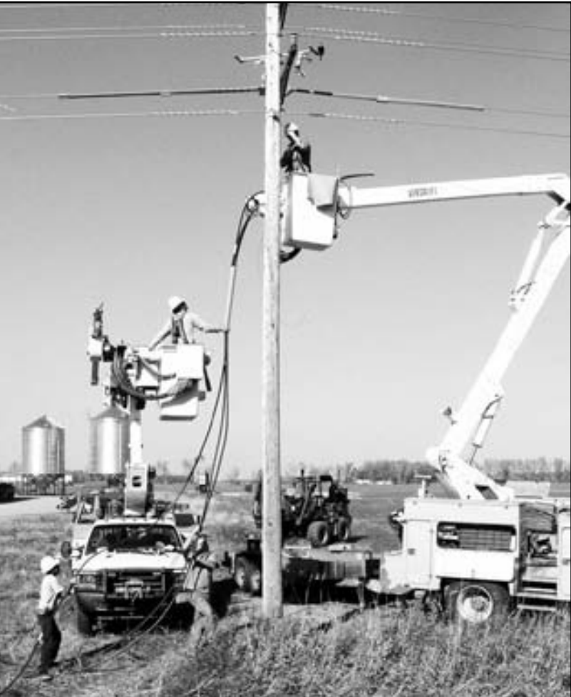
The line construction crew work to bring the underground wire up the three phase riser pole. Any pole that has underground wire run up the pole and terminated is considered a riser pole.
