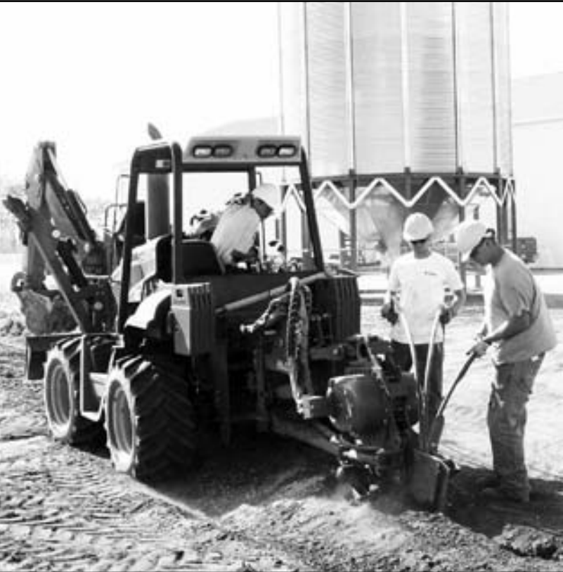
Roger Valley, operating the cable plow, Brett Knott and Jordan Gervais are installing underground wire for a three phase grain handling setup. Knott and Gervais guide the three underground wires through the plow shoe as the wire is buried. The three wires were strung out prior to the plowing.
