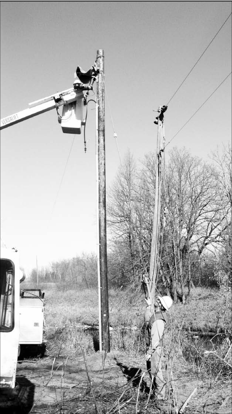
Once the phase wire has been attached to the new pole, linemen use a hoist to pull proper tension on the new pole prior to securing the guy wire.
