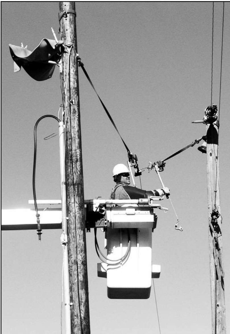
Schmitz uses two ratchet hoists to transfer the phase wire from the old pole to the new pole. The line remains energized in order not to interrupt electric service to member's accounts up-line.
