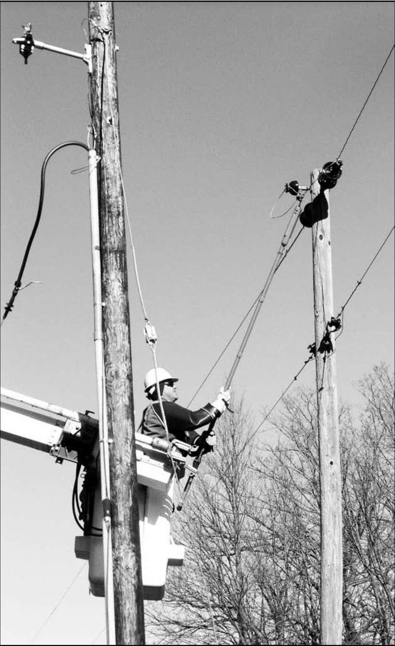
Troy Schmitz uses a shotgun (insulated fiberglass) stick to remove a hot-tap to open the section of overhead line that is being replaced with underground cable.
