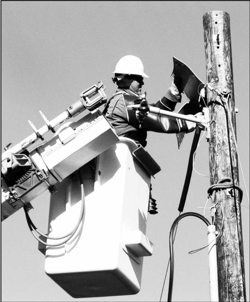
Schmitz places a rubber blanket over the phase wire prior to making the underground cable connections. The blanket and rubber gloves and sleeves Schmitz is wearing protects him from different potentials and the energized wire.
