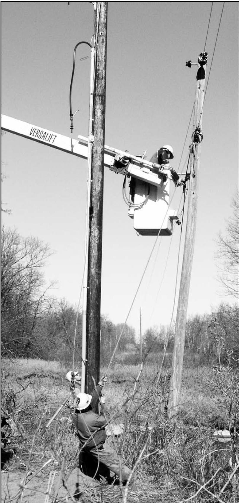
Linemen use a handline to drop the neutral wire, which crosses the river, from the existing pole. It will be re-attached to the new underground riser pole.
