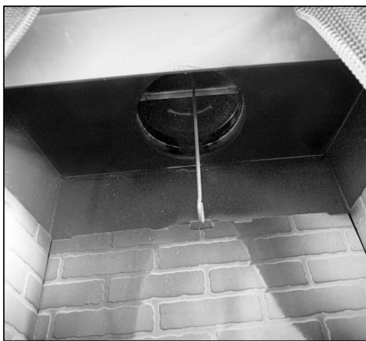
Open the fireplace flue when logs are burning to let smoke and heat out. But remember to close it when not in use to keep conditioned or heated air inside.
