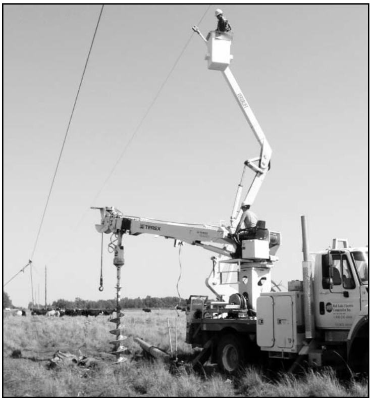
The dry land conditions allowed line personnel to get cooperative vehicles into a pasture that under normal conditions would have required the use of a track digger. Several poles in this pasture were changed or reset.
