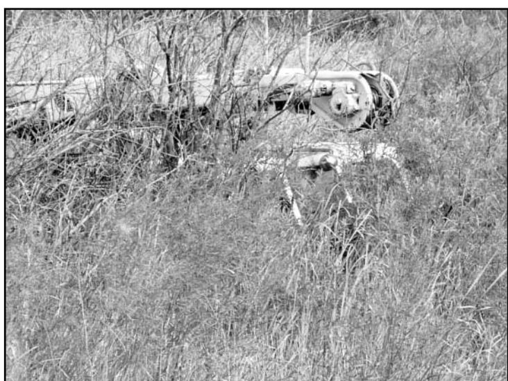
Red Lake Electric line personnel travel through the brush and swamp with the track digger to change out poles in the swamp that in most normal years would be standing in water.
