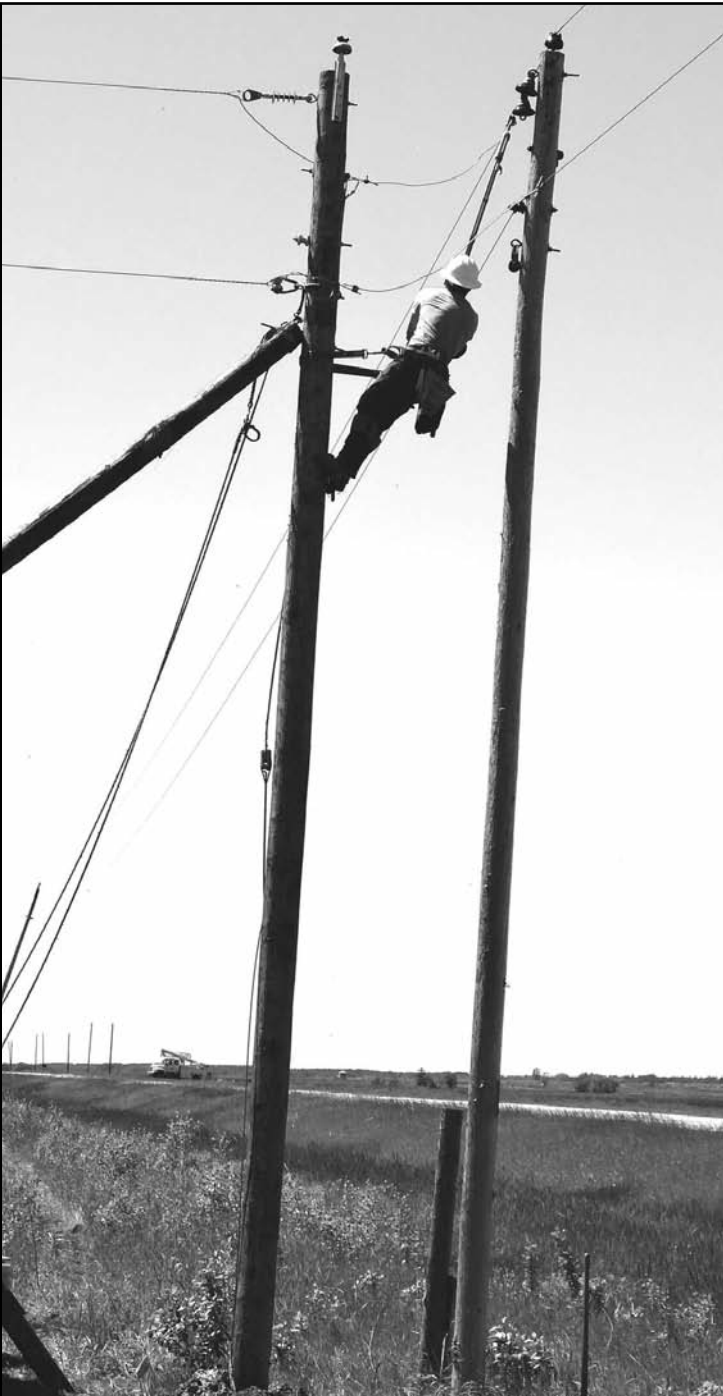
This view shows the old line, which was leaning towards the road, and the new line constructed next to it. Foreman Casey Thronson is shown disconnecting the tap line to one of our members in order to attach it to the new line.
