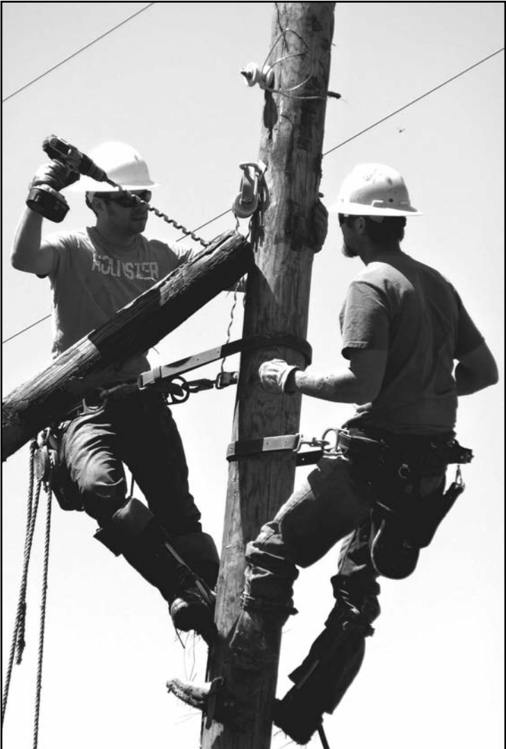
RLEC employees Casey Thronson and Brett Knott are shown securing the push pole to the new line pole.
