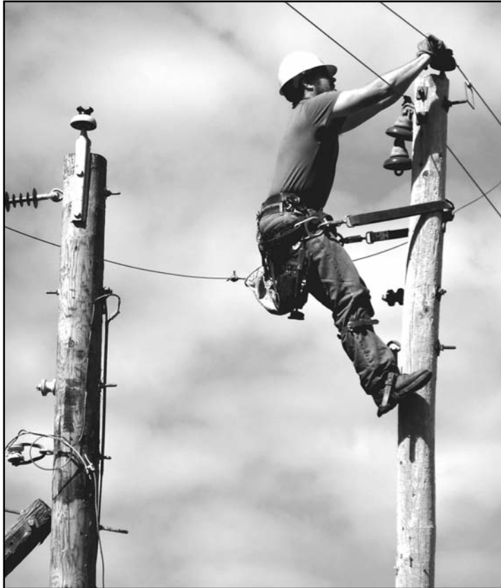
RLEC lineman Aaron Derosier is untying the wires on the old line.
