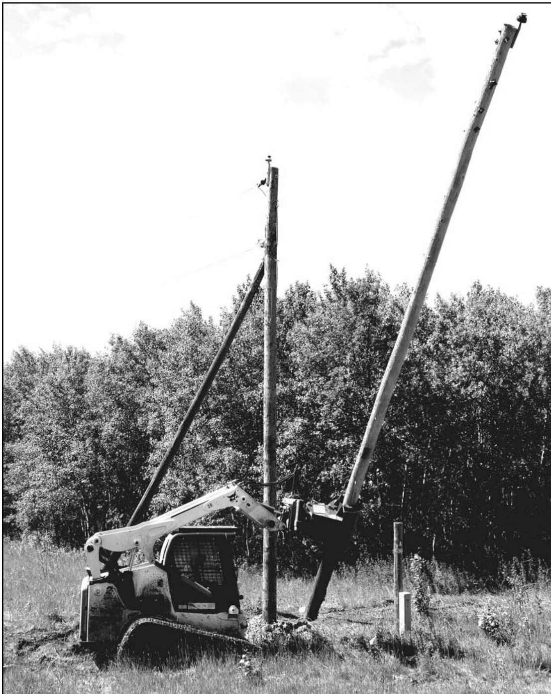
One of the new pieces of equipment, a Bobcat skid steer, is being used along with a pole clamping attachment to remove the old poles.
