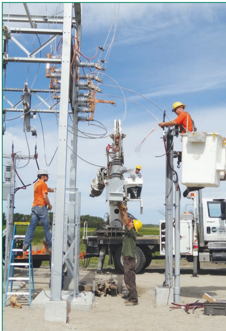
Red Lake Electric Cooperative line personnel work to set a breaker in the Gentilly Creek substation. Branden Narlock, lineman in the bucket, works on terminating underground wire on a riser in the substation. The Gentilly Creek substation was energized Sept. 17 and serves 223 cooperative members in Polk County.
