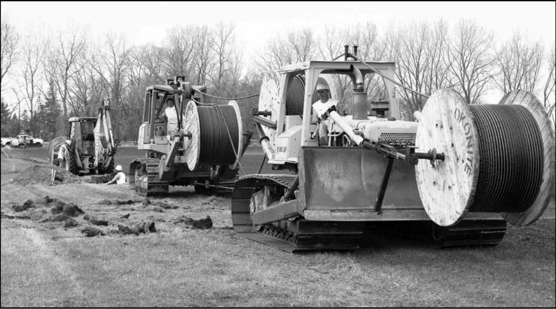
Trudell Contracting of Warren plowed 4 1/2 miles of three phase underground line to be used to distribute the electricity from the Gentilly Creek substation. This line runs along Polk County road 11 and serves Red Lake Electric members east of Crookston.
