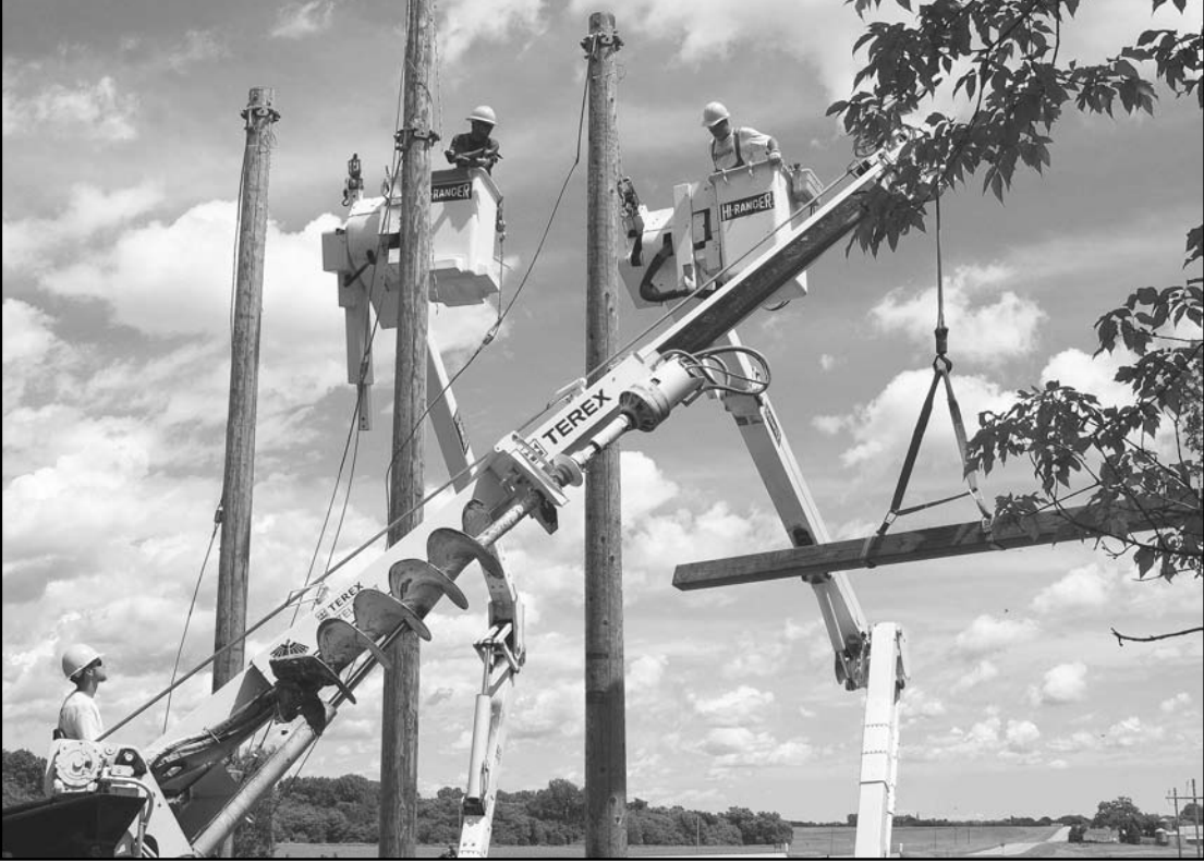
Red Lake Electric line personnel work to construct one of the riser structures for the overhead line crossing of the Red Lake River by the Gentilly bridge.
