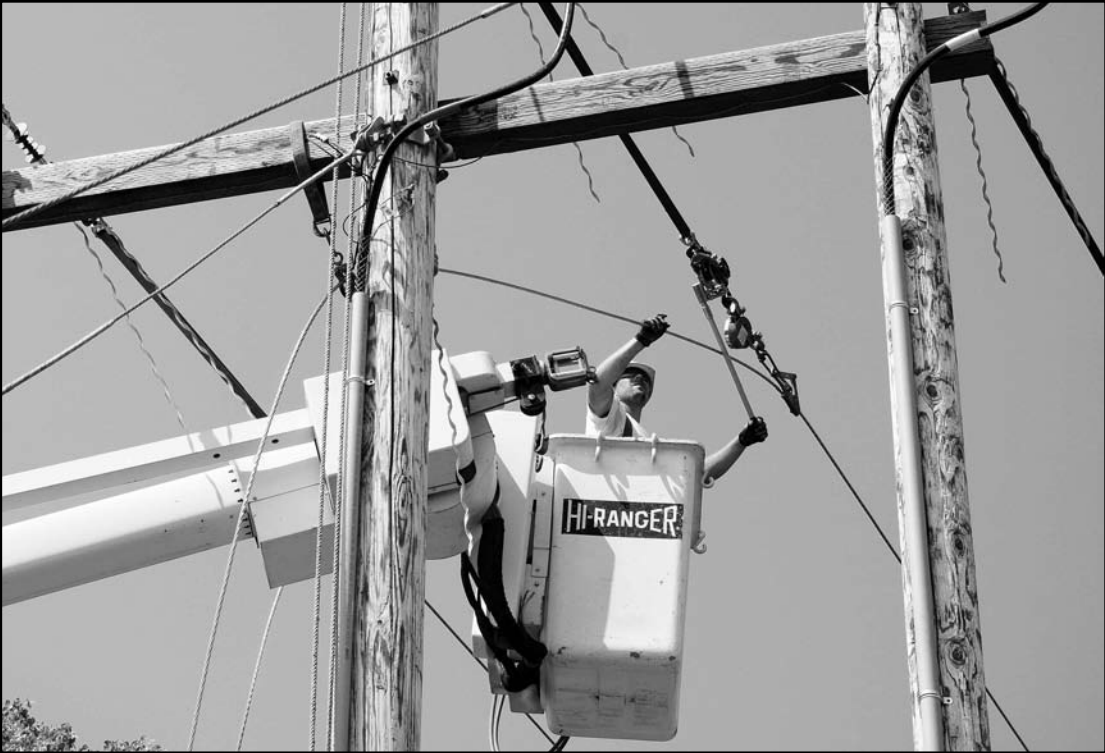
Aaron Derosier, apprentice lineman, uses a web hoist and dynamometer to pull the wire into proper sag over the Red Lake River along side the Gentilly bridge. The dynamometer measures the tension on the wire.
