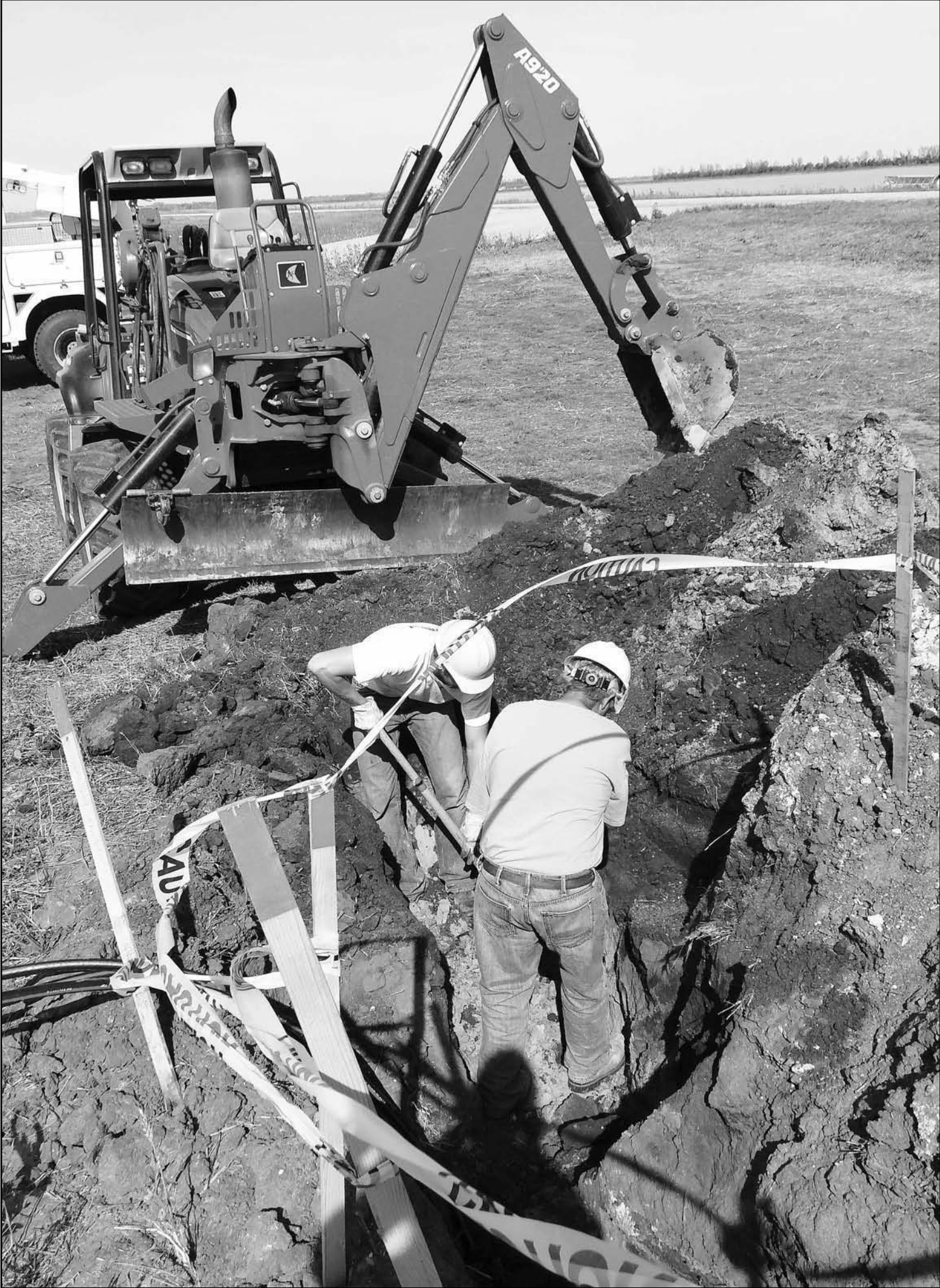
Brett Knott (L), lineman, and Alan Cota, retired crew foreman, dig to expose existing underground cable so it can be spliced to the new cable coming out of the Gentilly Creek substation. Infrastructure improvements associated with the new substation spanned throughout the summer for Red Lake Electric line crews.
