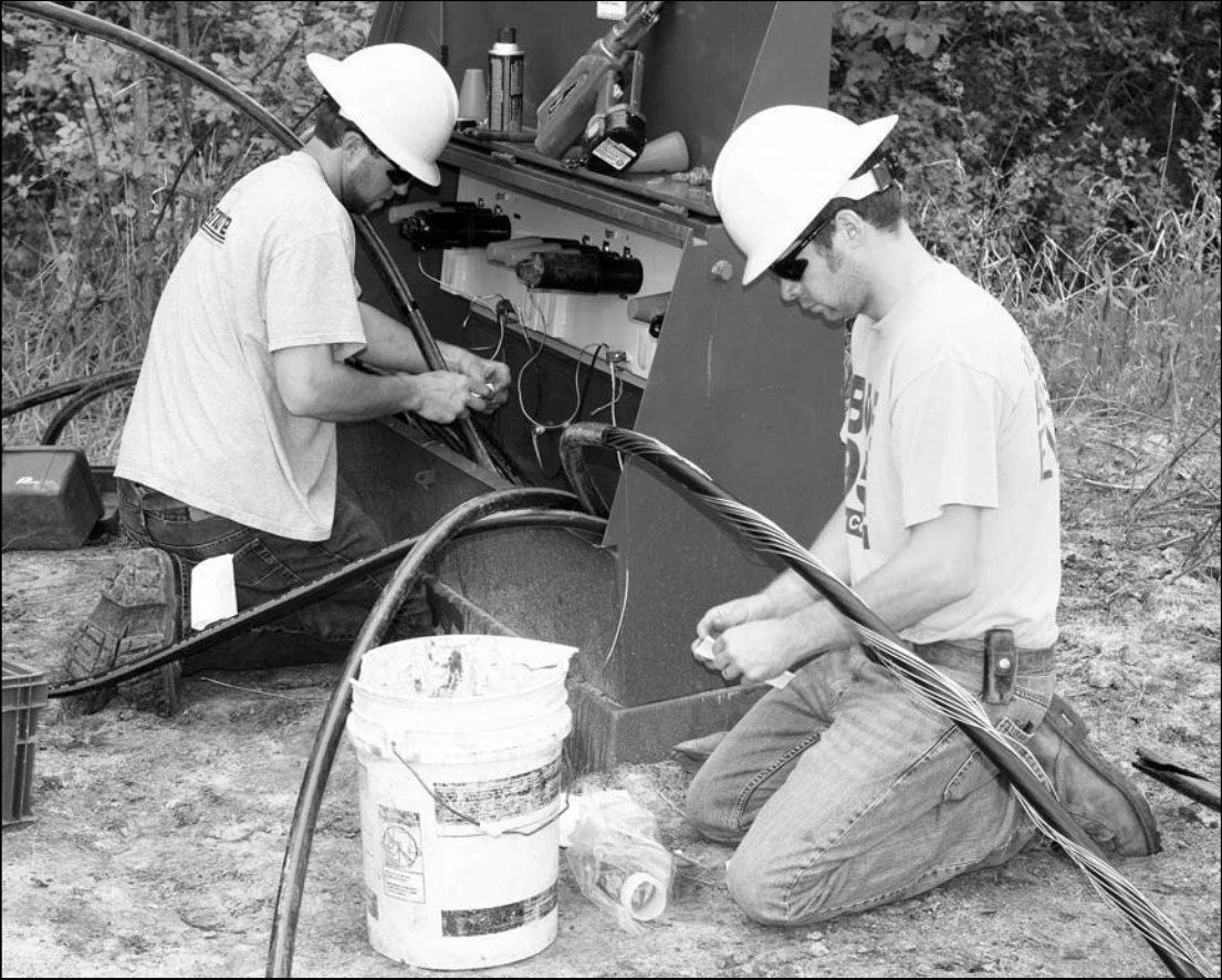
Sam Pahlen (L), apprentice lineman and Casey Thronson, crew foreman, with Red Lake Electric, work to complete the terminations in one of several junction boxes as part of the new three phase underground line along Polk County road 11 west of Gentilly.
