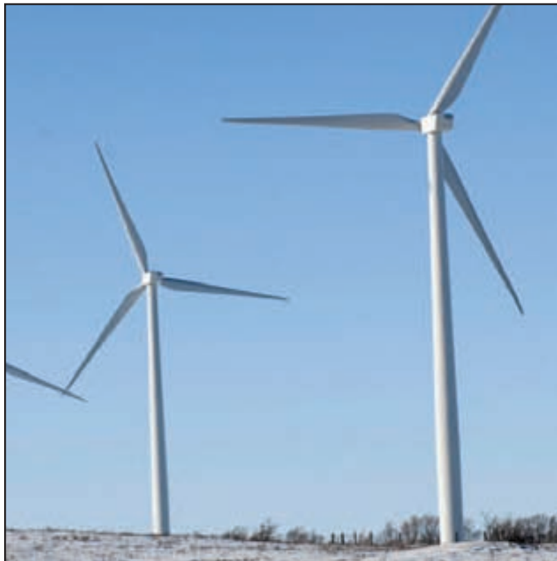
The Ashtabula 1 wind generator farm is located in Barnes County, ND, and can produce 148.5 megawatts from ninety nine 1.5-megawatt GE turbines. Each turbine is more than 260 feet tall from the ground to the center blade hub. The site began commercial operation in 2008. The site is operated by a subsidiary of NextEra Energy Resources.
