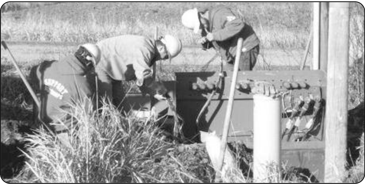
Nearly a 1/2 mile section of three phase underground was replaced SE of Goodridge. The cable was plowed by Trudell Contracting of Warren and the terminations were done by Red Lake Electric line workers. Terminations are being made in a three phase junction cabinet by (L to R) Jordan Gervais, Brett Knott, and Sam Pahlen.
