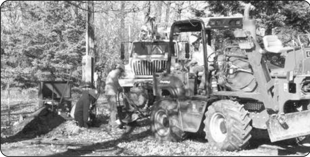
Red Lake Electric Cooperative line crew employees (L to R) Brett Knott, Casey Thronson, and Roger Valley work to convert an overhead service to an underground service. The change was made to eliminate the need to continually trim spruce trees near the overhead line. The conversion was cost shared with the Cooperative member.
