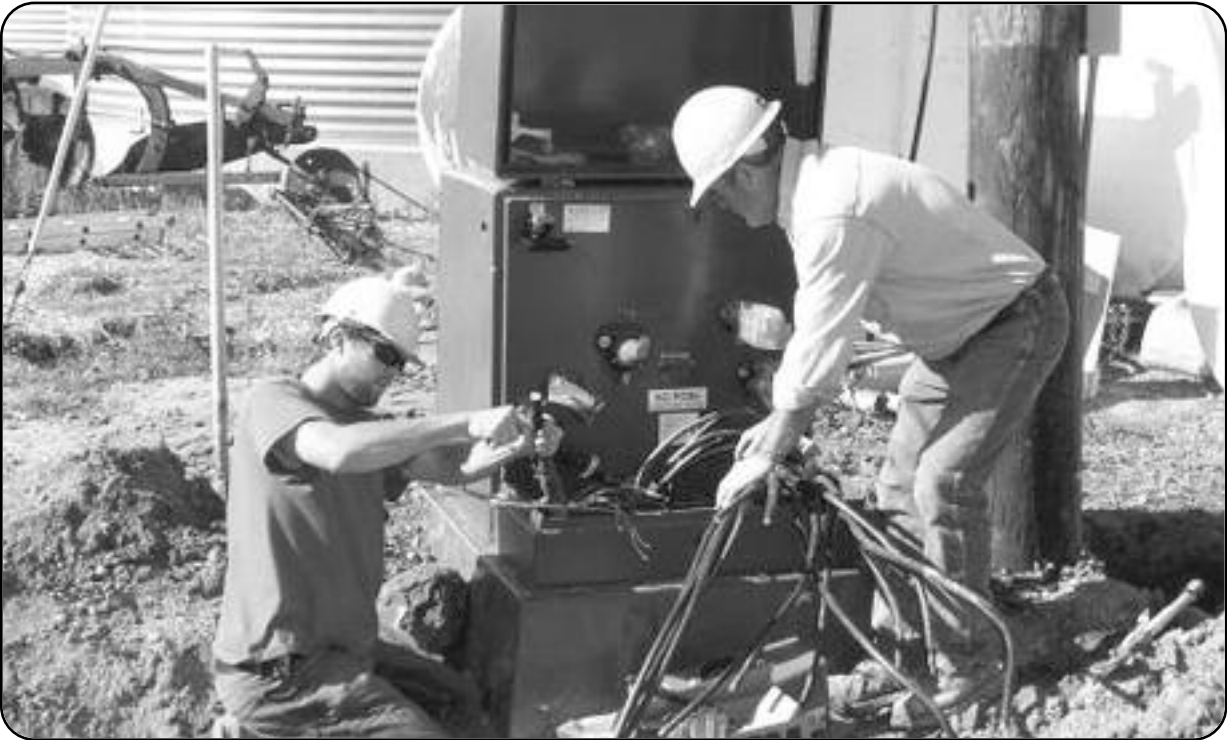
Sam Pahlen, seasonal line worker, and Mike Wavra, lead lineman, work to terminate wires in an underground transformer cabinet. This service needed to be upgraded for additional grain handling/drying equipment. The service was supplied by an overhead transformer and was changed to an underground transformer.
