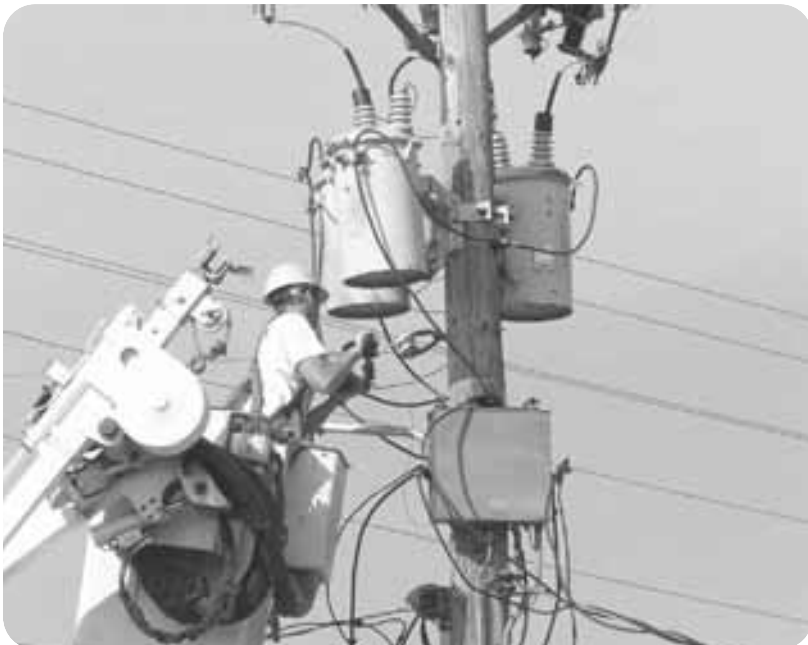
Brett Knott makes the final connections on the service pole for Evans Scrap and Steel. Evans along with a few other members were without electrical service for a few hours while the transition work was being done. All other members continued to receive electric service during the transition as feeder lines were switched and back fed from other directions.
