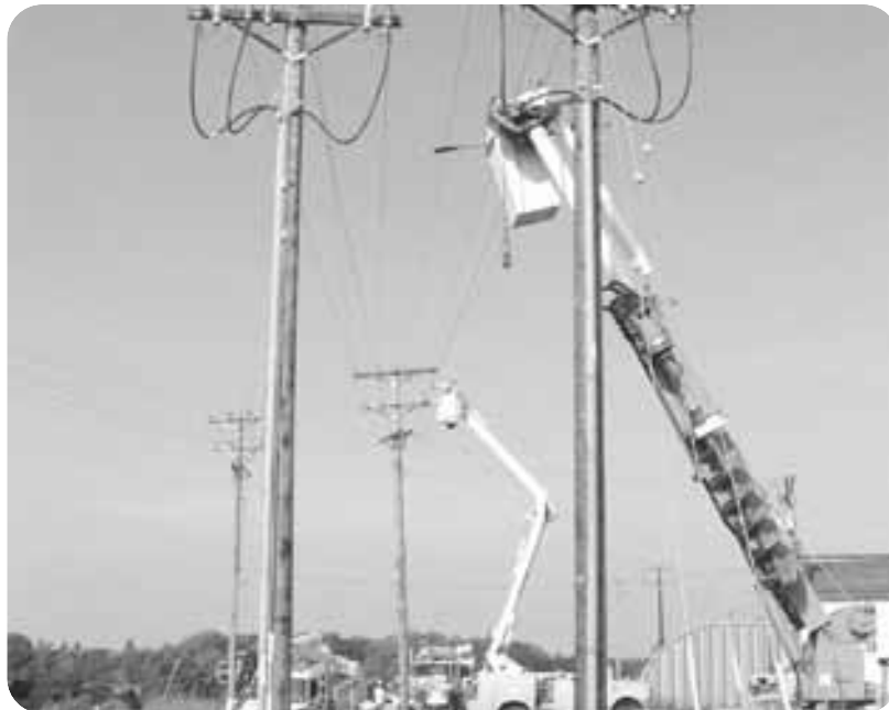
The two overhead circuits separate and terminate on two different riser poles where the overhead wires are connected to underground cable. The right structure is for service to members immediately NW of Thief River Falls in four sections of North Township. The left structure is for service to members in six different townships west of Thief River Falls up to 18 miles away.
