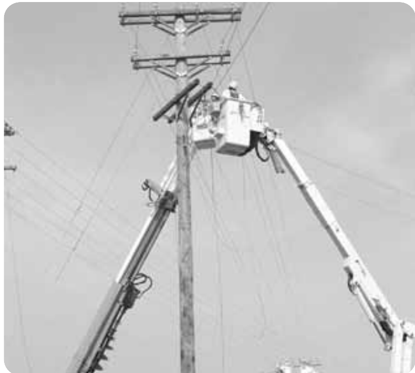
Line personnel Dick Gervais, left, and Brett Knott do work on one of the new double circuit structures. The structure also serves as the take off for the three-phase service for Evans Scrap and Steel.
