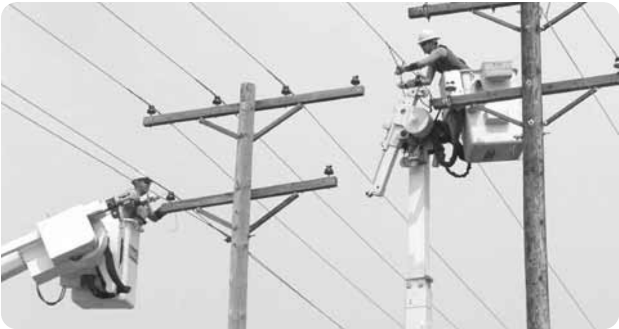
Once the poles were set for the new double circuit line Red Lake Electric linemen Alan Cota, left, and Casey Thronson work to untie the wires from an old structure and transfer them to a new structure.
