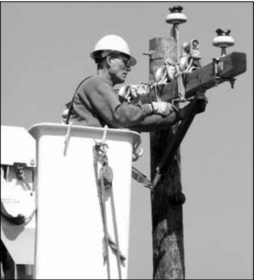
A Red Lake Electric construction crew works to set a new pole east of the Schafer farm. The existing single phase overhead line was converted to three phase. The two linemen in the bucket trucks hold the existing wires out of the way using the jibs at the end of the booms.
