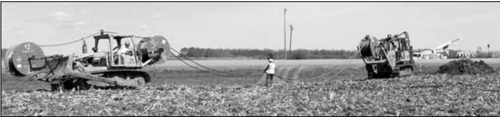
Trudell Contracting plowed in three phase underground cable on the Walker farm north of Red Lake Falls. Approximately 1/2 mile of underground was part of Otter Tail Power's two-mile re-route of line.
