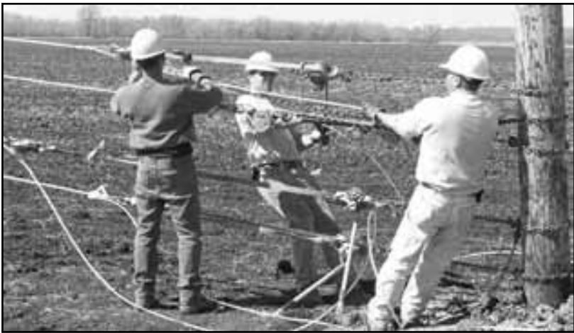
Following the stringing of the wires, the wires need to be pulled to the proper tension. This is accomplished using web hoists and dynometers. The dynometers record the tension on each wire. Red Lake Electric employees pulling the wires are, from left, Ira Cota, Aaron Derosier and Dick Gervais.
