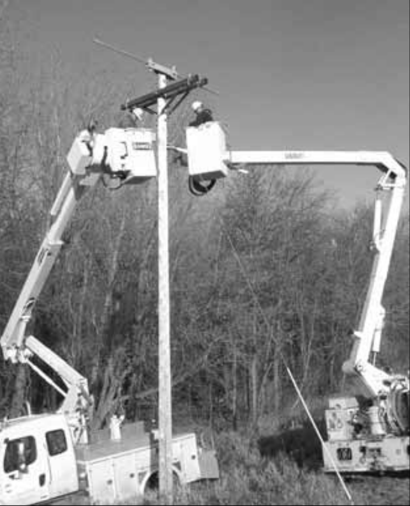
Red Lake Electric employees Troy Schmitz, left, and Dick Gervais work to convert a single phase pole to a three phase structure east of the Halvorson farm northwest of Red Lake Falls. The west end of the three phase tie-line was connected to the three phase overhead line from the Huot substation which is just east of the Halvorson farm. Note the rubber hoses and rubber blanket that protect the linemen from the existing phase wire which remains energized while they work.
