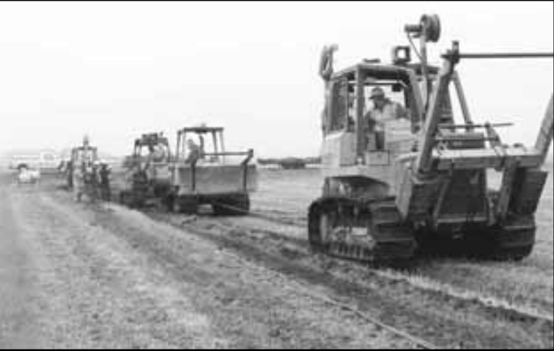
In October of 2009, Trudell Contracting of Warren plowed in 1-1/2 miles of three phase underground cable west of the Schafer farm northwest of Red Lake Falls. It is part of a three phase tie-line between the Terrebonne and Huot substations. Two crawlers were needed to pull the plow through the heavy soil.
