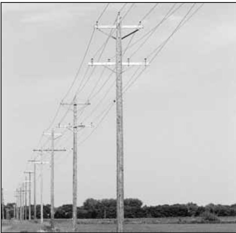
This is the completed double circuit line north of Red Lake Falls. Otter Tail Power's three phase feeder line for St. Hilaire is on the top of the structures. Red Lake Electric's three phase tie-line is on the lower crossarms. This new line will provide many years of service for both Otter Tail Power and Red Lake Electric customers.
