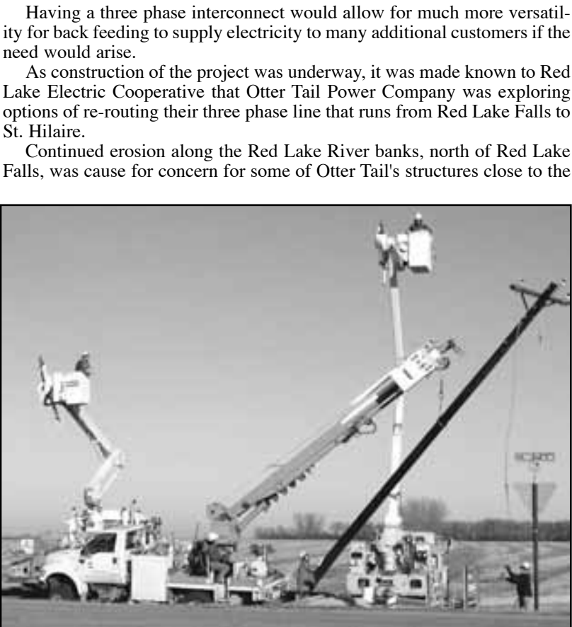
A Red Lake Electric construction crew works to set a new pole east of the Schafer farm. The existing single phase overhead line was converted to three phase. The two linemen in the bucket trucks hold the existing wires out of the way using the jibs at the end of the booms.
