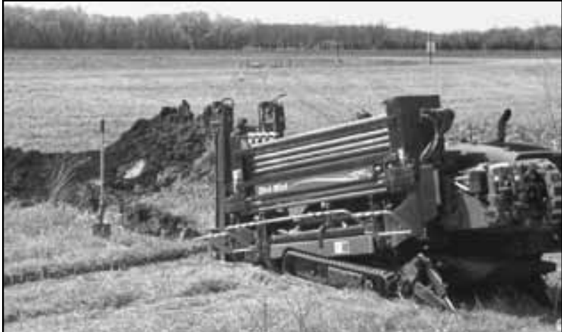
Above: Trudell Contracting uses a boring machine to bore under Red Lake County Highway 19. A hole was bored into the pit on the other side of the roadway. The underground cable was hooked to the bore pipe and pulled under the highway, causing no disruption to the asphalt-covered road.
