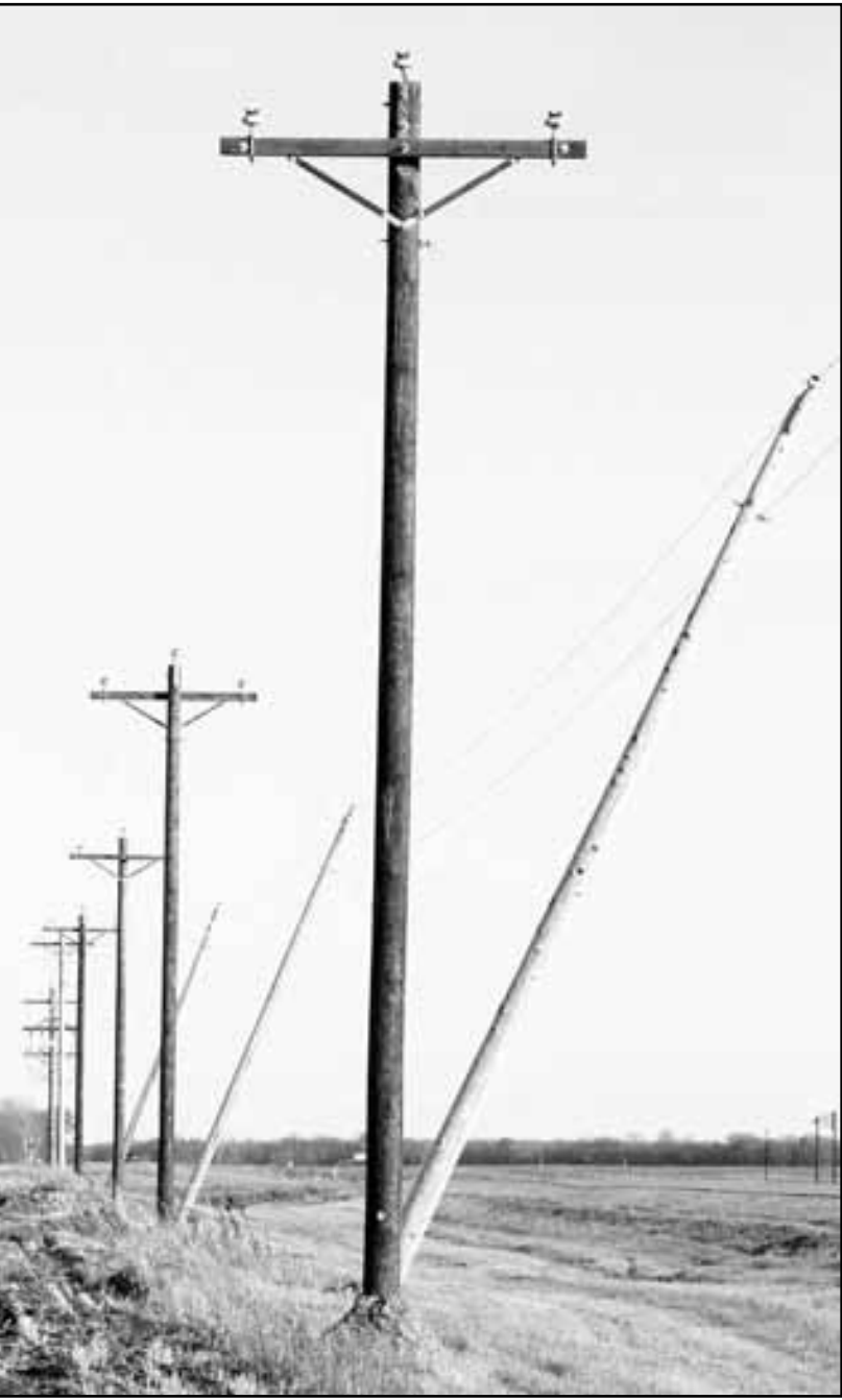
Above: The existing single phase poles were re-set at an angle to allow for the new three phase structures to be set in place. This work is all part of the three phase tie-line between the Terrebonne and Huot substations.
