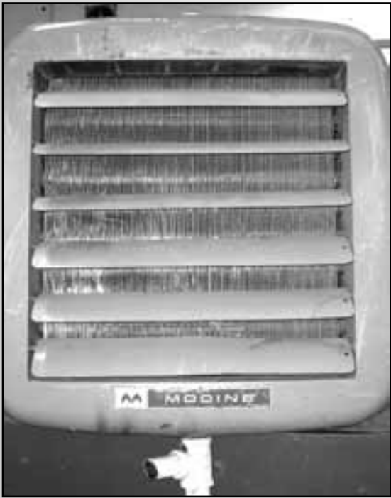
Lot 1: Modine steam or hot water unit heater, 10 years old. 1/6 HP 115V fan motor.
