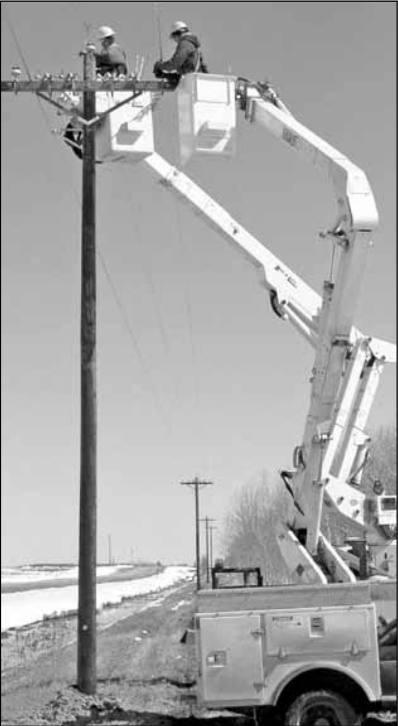
Following the setting of poles for the new overhead line, wire was strung and tied in on the insulators.
