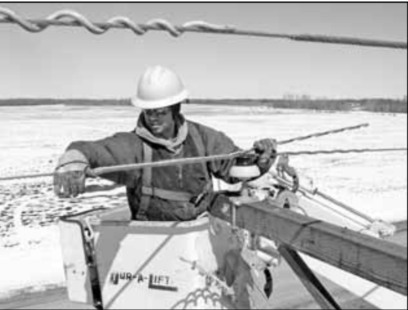
Casey Thronson, lineman, wraps the wire with armor rod prior to the wire being tied to the insulators. Armor rod helps to prevent breakage of strands of wire due to movement and/or vibration of the wire.
