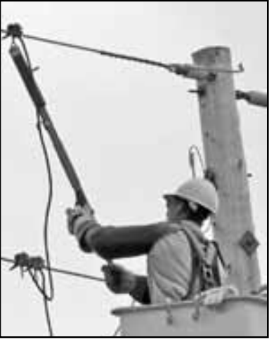
Ira Cota, lineman, uses a shotgun stick (insulated fiberglass stick) to install grounds, grounding out one set of wires leading to the pole that is to be changed. The leads to these wires have been cut allowing the wires to be de-energized and isolated. The grounds are installed to make sure the wires remains "dead" during the changeout.
