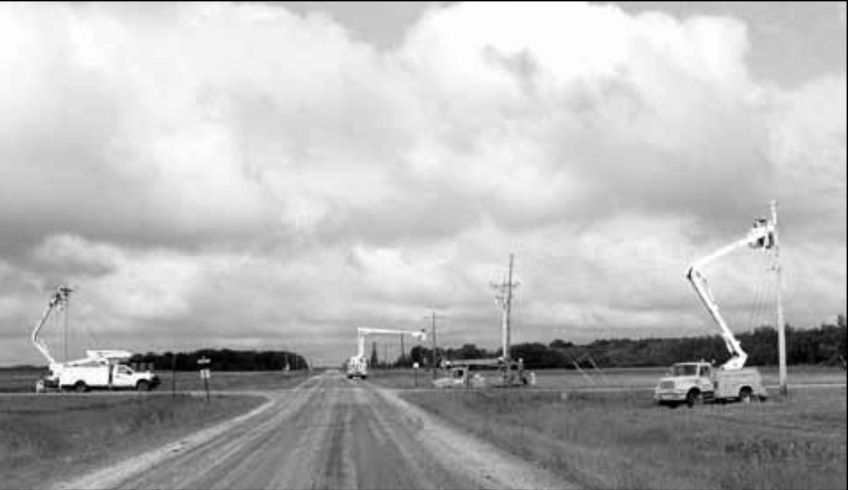
Line crews work on all three sides of a three phase corner pole to isolate the corner pole taking it out of service for replacement. It is the last major task associated with the line conversion project. There is a breaker pole that will also be taken out of service as a new one had been constructed.
