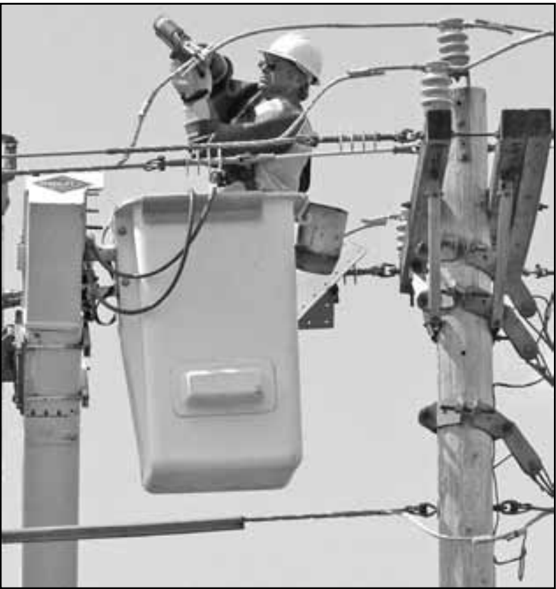
Once the replacement of the three phase corner pole has been completed, Dick Gervais uses a battery operated crimp tool to reconnect one set of wires that had previously been cut. He is equipped with rubber gloves and sleeves as the connections are being made to "hot" or energized wires.
