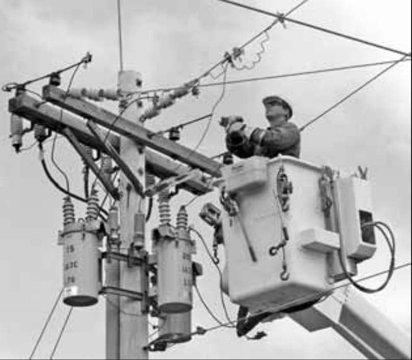
Troy Schmitz, lineman, begins to remove the hardware from the old breaker pole as it is being retired. With this being a three phase line there is one breaker, or oil circuit recloser, for each phase.
