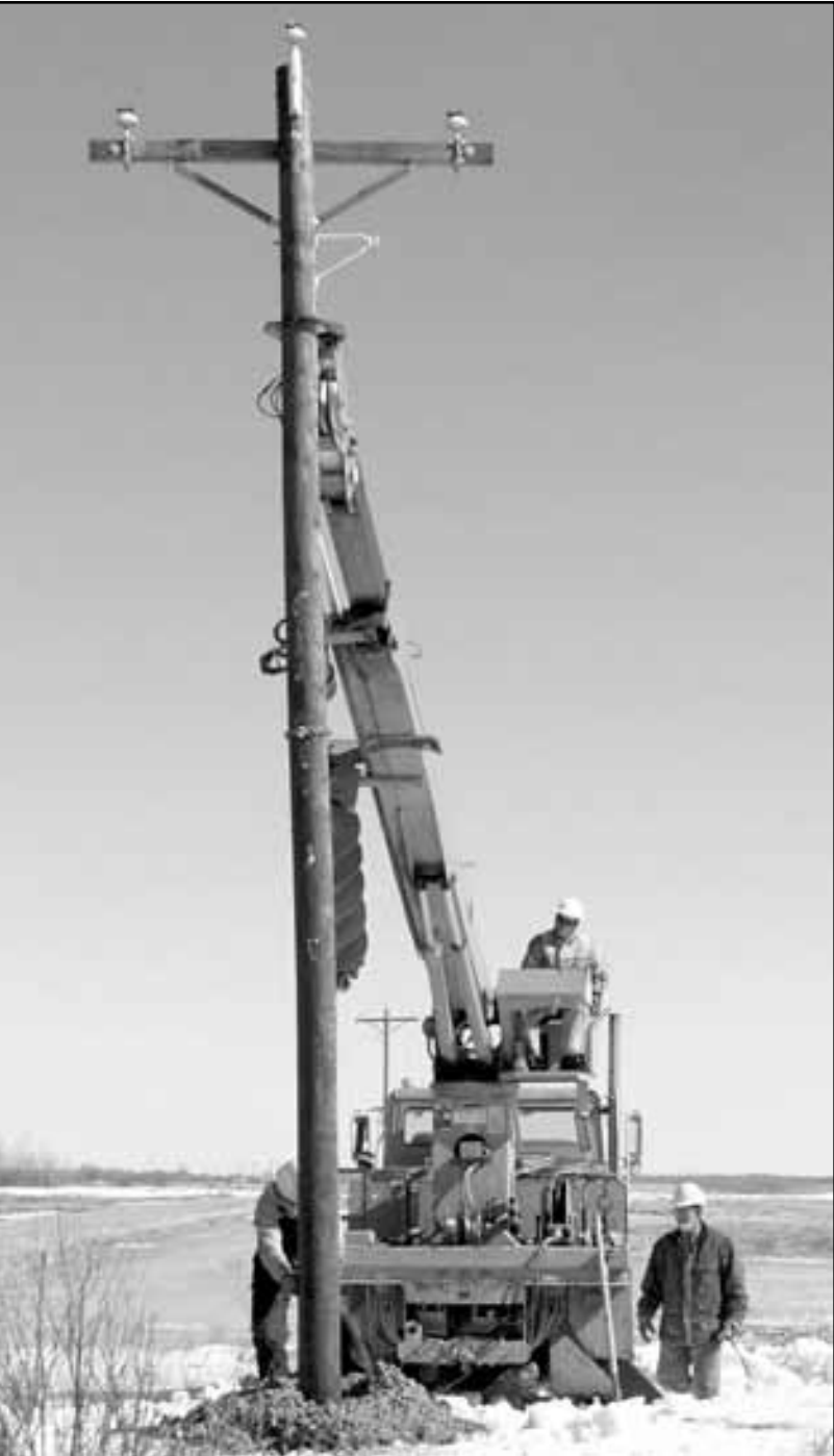
Conversion of an underground line to overhead, northeast of Viking, began in March. Members in the area experienced an outage due to another cable failure which prompted the conversion project to begin. Many of the three phase poles were set in less than ideal conditions due to snow and water.
