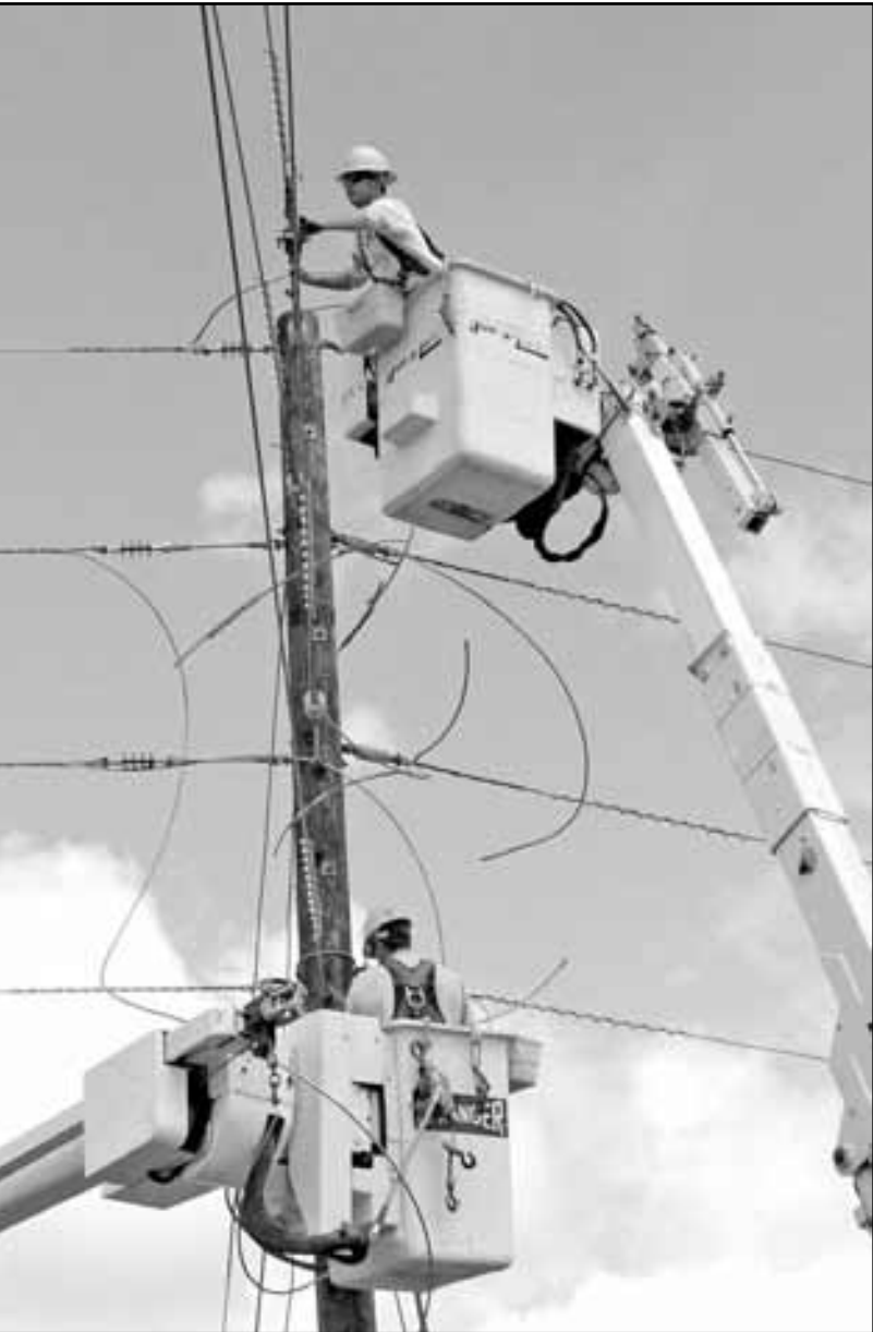
Casey Thronson, top bucket, and Troy Schmitz work to finish dead ending the three sets of three phase wires that attach to the new three phase corner pole.
