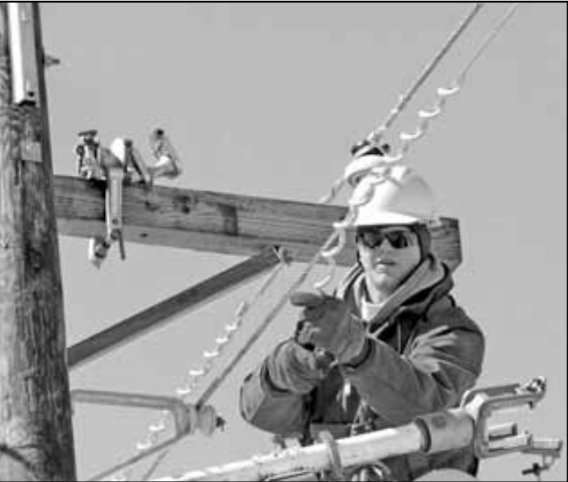
Brett Knott, apprentice lineman, installs vibration dampners on the wires. Vibration dampners are used to help reduce wire movement due to wind or ice build up. Reducing wire movement helps to reduce the loosening of hardware on the structures.
