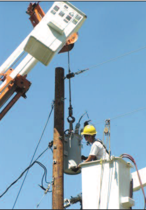
Brett Knott, apprentice lineman, guides the transformer onto the mounting bolts of the transformer pole at the Nelson residence northwest of St. Hilaire. The transformer is raised with the winch of the digger truck.
