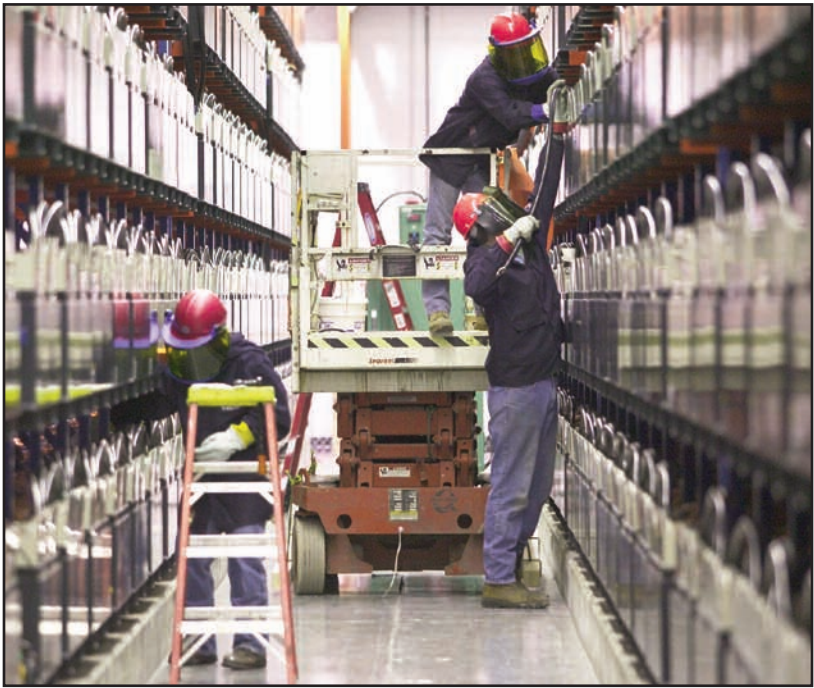
Golden Valley Electric Association, based in Fairbanks, Alaska, uses the world's most powerful nickel-cadmium battery to hedge against power outages. When needed, the 13,760-battery cell system can provide 27 megawatts of power for 15 minutes. Source: Patrick Endres/Alaskaphotographics.com
