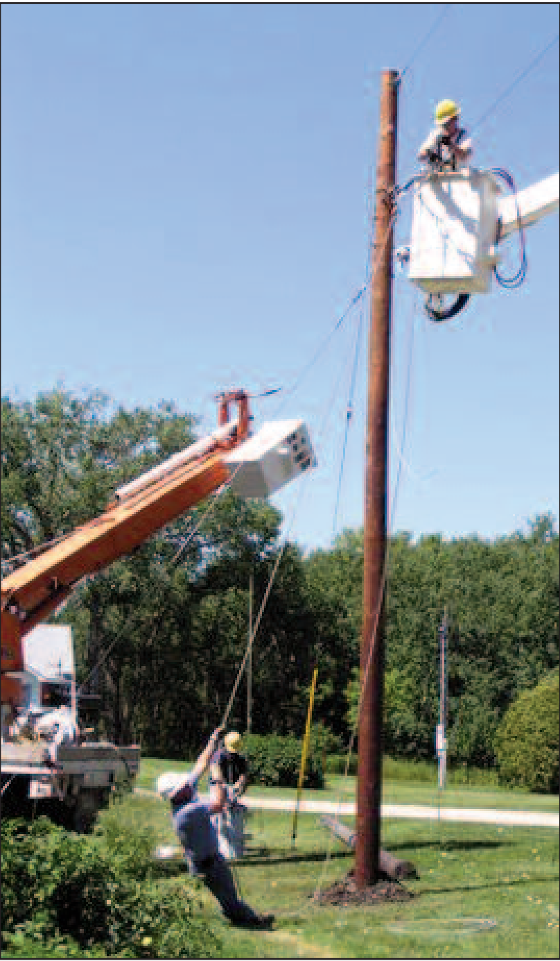
Dick Gervais, front left, uses a handline to raise the primary wires for the new transformer pole in the yard of Gary and Barb Nelson.
