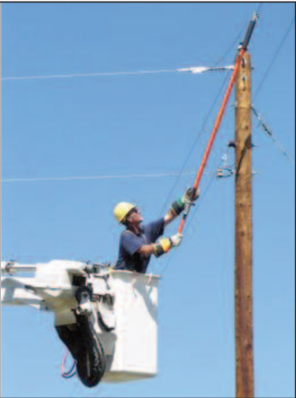
Once the electric service into the Nelson yard has been redone, the tap is connected to energize the service. Ira Cota, lineman, uses an insulated fiberglass stick to connect the hotline tap. The relocation of this take-off pole along County Road 15 northwest of St. Hilaire was cause for the Nelson service to be redone.
