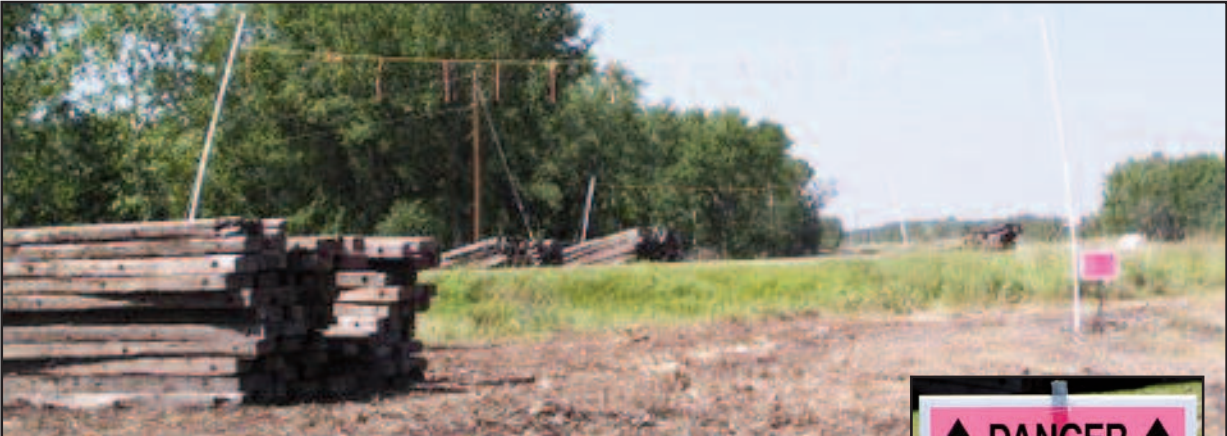
Above: Safety is a big concern for pipeline construction workers. Every overhead power line crossing is marked for the construction workers. White plastic poles with a rope and orange flag are set on each side of every overhead crossing. The piles of timbers in the picture are used for bridging material at every ditch crossing. Inset: Also at each overhead powerline crossing, pipeline construction workers are reminded of the overhead lines by a warning sign.
