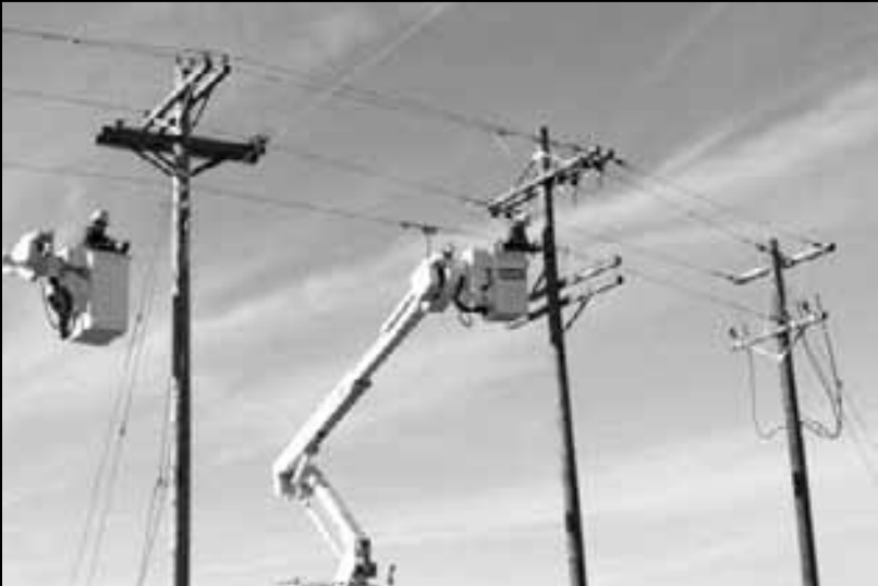
Work nears completion on the new take-off pole and breaker pole as linemen work to make final grounding connections.
