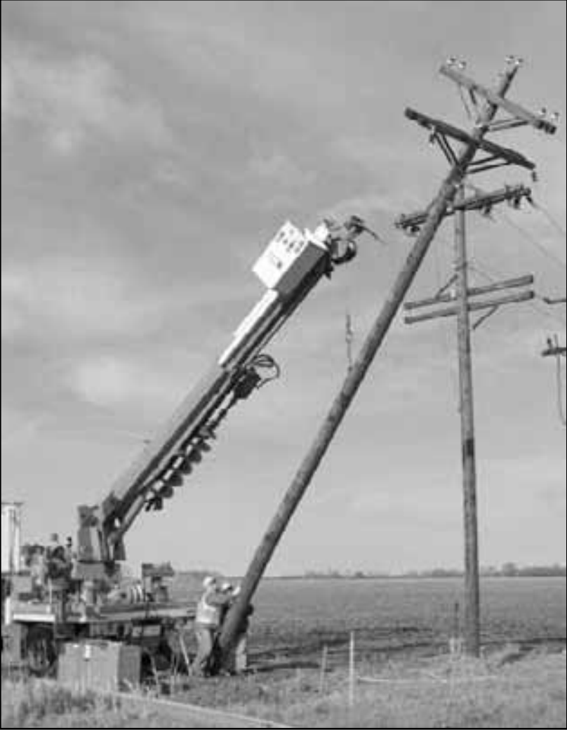
A new corner/take-off pole is lifted into place on the west side of County Road 5. It is a 40-foot pole and has a cost of $400 for just the pole.
