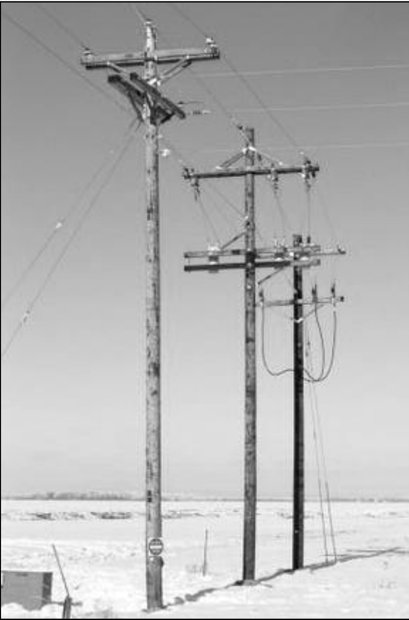
Everything is complete on the new take-off pole, breaker pole and riser pole for the three-phase underground just north of Oklee.
