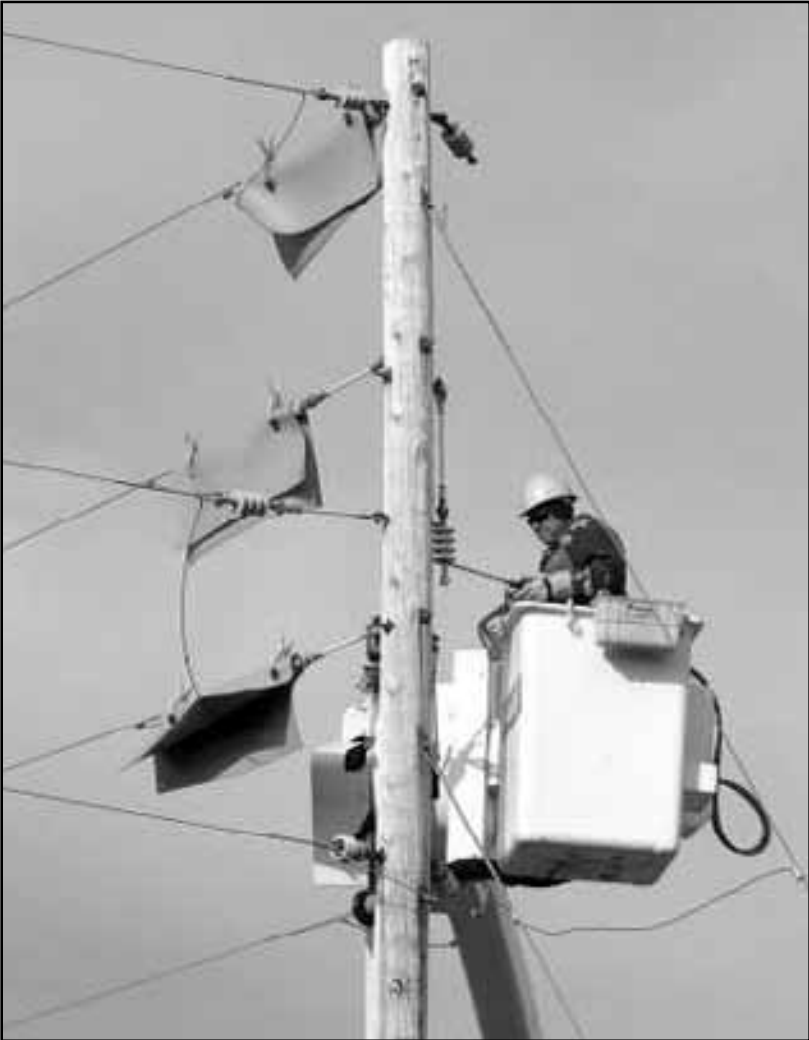
Alan Cota, lead lineman, works to install epoxilators on a corner pole on the south side of the new take-off pole and breaker pole. Insulated blankets are used to cover up hot wires to help avoid any accidental contact.
