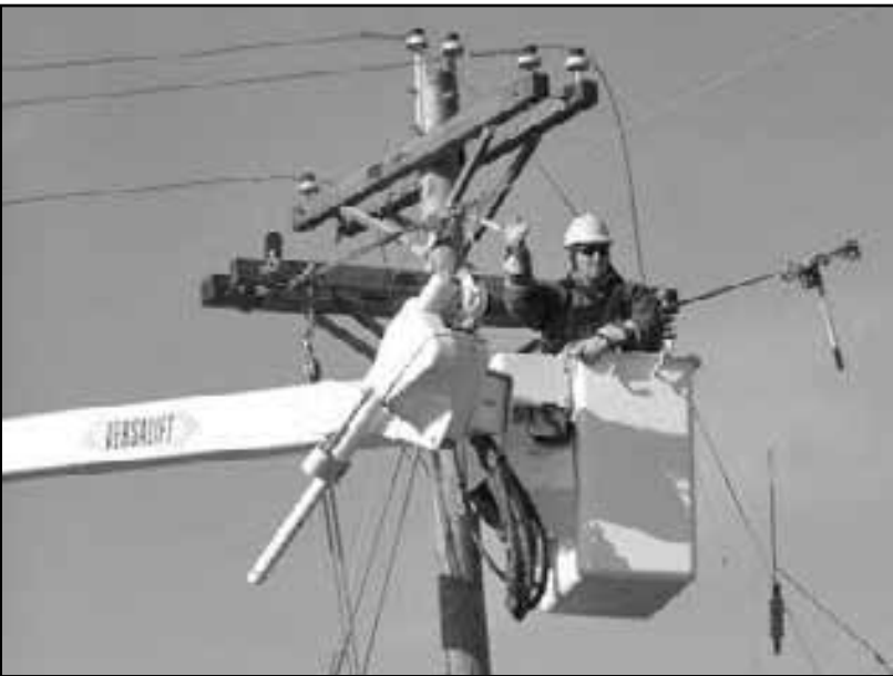
Troy Schmitz, lineman, uses coffin hoists to bring the two-phase overhead wires into proper height and tension onto the take-off pole. The wires cross County Road 5 going east.
