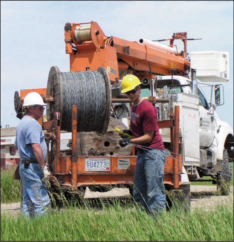
Dick Gervais, left, and Brett Knott reel up the old amerductor using a wire winder on the trailer. The amerductor wire has served its purpose for about 60 years but now will be sold as scrap.
