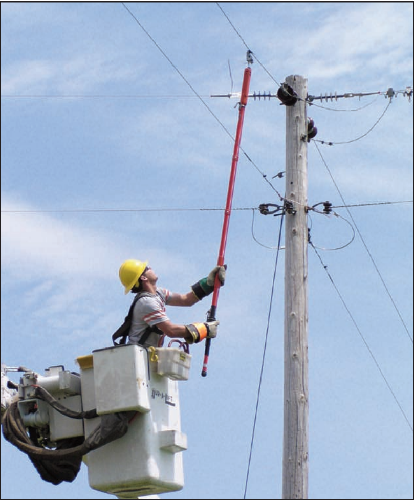
Tying in of the new wire has been completed. Casey Thronson uses a shotgun stick (fiberglass insulated stick) to attach the hot tap (clamp) to the phase wire to re-energize the line.
