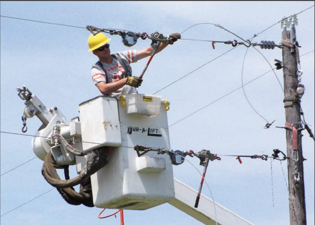
Once the wire has been set on all the insulators on the poles, Casey Thronson, lineman, uses ratchet hoists and a dynamometer to pull the wires into proper tension. Factors that determine the tension include wire size, pole span and ambient temperature.
