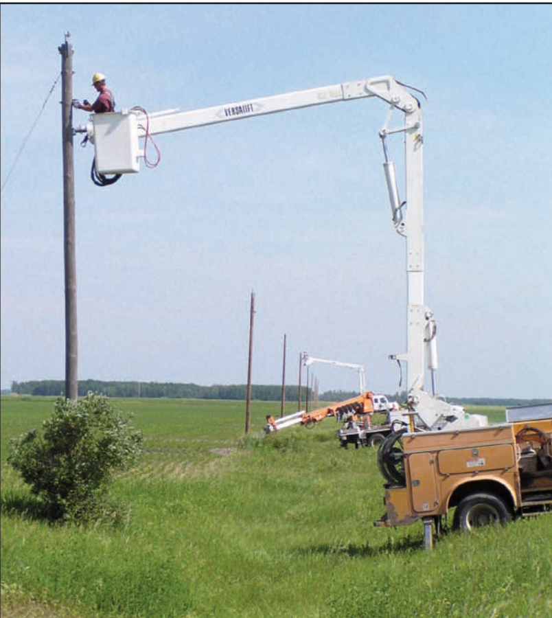
Red Lake Electric Cooperative line crews work to upgrade a single-phase line northeast of Plummer. Lineman Ira Cota, in the foreground bucket, unties the amerductor wire allowing it to fall to the ground.
