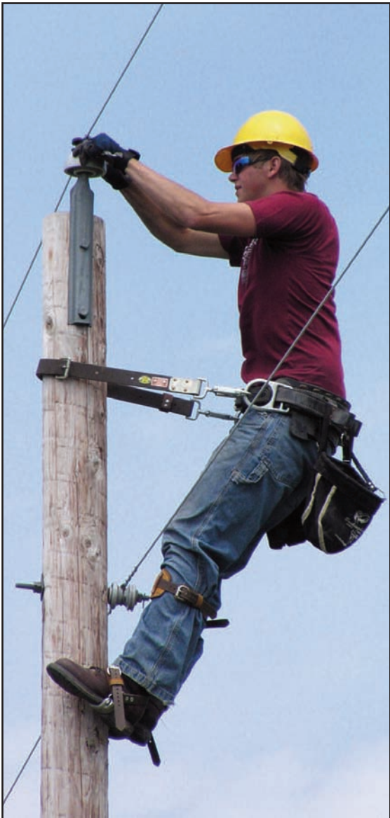
After the new aluminum wire has been pulled to proper tension, preformed ties are used to secure the wire to the insulators. Brett Knott, apprentice lineman, ties the conductor wire to the pole-top insulator.
