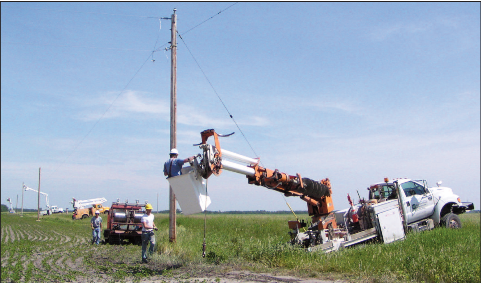
New aluminum wire for the line upgrade is strung out with the reels of wire on the back of the Bombardier. Dick Gervais, crew foreman, in the bucket, prepares to lift the wire up onto the pole.
