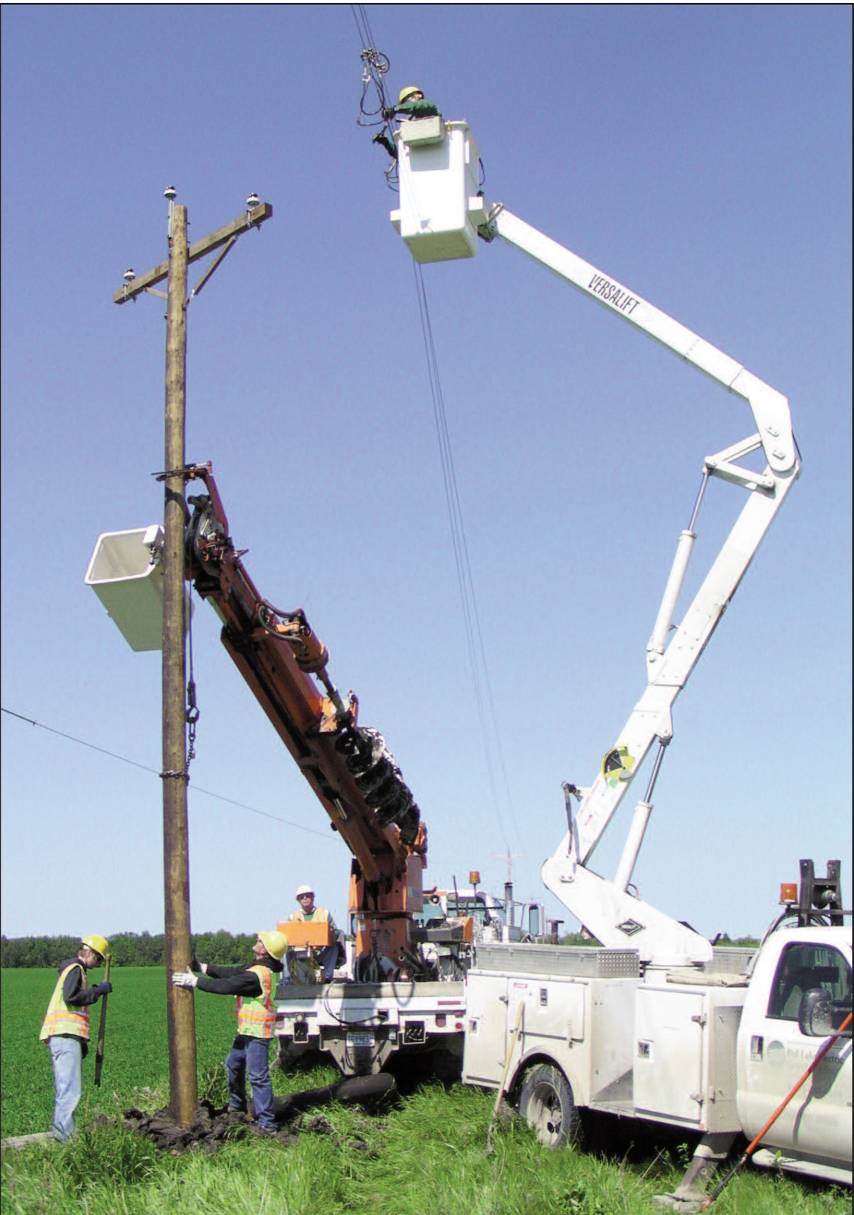
Wires are lifted and held out of the way with the jib at the end of the boom of the bucket truck while a new three-phase pole is set by a line construction crew. In addition to Troy Schmitz, crew members are Dick Gervais, crew foreman; Ira Cota, lineman; and Brett Knott, apprentice lineman.
