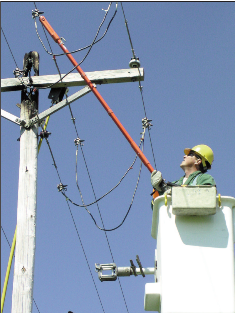
With the line de-energized, Troy Schmitz, lineman, uses a shotgun stick to attach grounds on all the wires on the three-phase pole before the pole is changed out. The grounds are used as a safety precaution in case of any backfeed on the lines.
