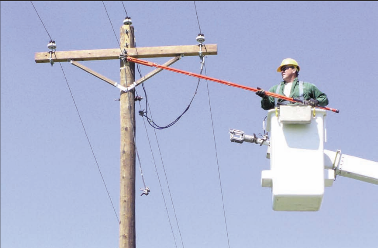
Once the work is complete, Troy Schmitz removes the grounds from the wires so the line can be re-energized. The change-out of the pole resulted in about a one-hour electrical interruption for RLEC members in the Brooks/Oklee area.
