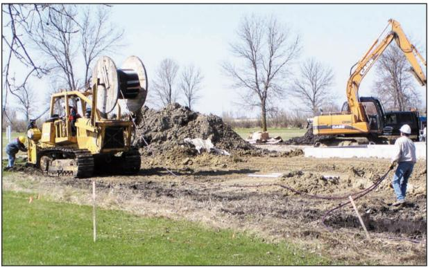
An underground service was installed for a new cell phone tower north of the football field at Oklee. The underground cable was plowed in by Garden Valley Telephone Company. It was a joint plowing since Garden Valley and Red Lake Electric's cables were plowed at the same time. Roger Valley, crew foreman, positions the cable ahead of the crawler while Casey Thronson, apprentice lineman, helps the cable down the plow chute at the back of the crawler.
