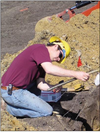
An underground service is constructed north of Red Lake Falls and has to be tied into an existing underground cable. The existing cable has been located, uncovered and cut open. Casey Thronson prepares the cut cable for an underground cable elbow, which will allow the cable to plug into a junction box.
