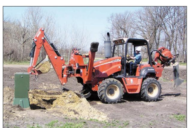
The underground work has been completed, the cable for the new service is energized and Roger Valley works to fill the splice pit.
