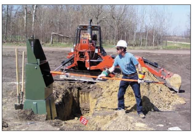
Once the cable splice has been completed, Roger Valley uses a shotgun stick (insulated fiberglass stick) to plug the underground cable elbows into the junction box placed at the splice pit.
