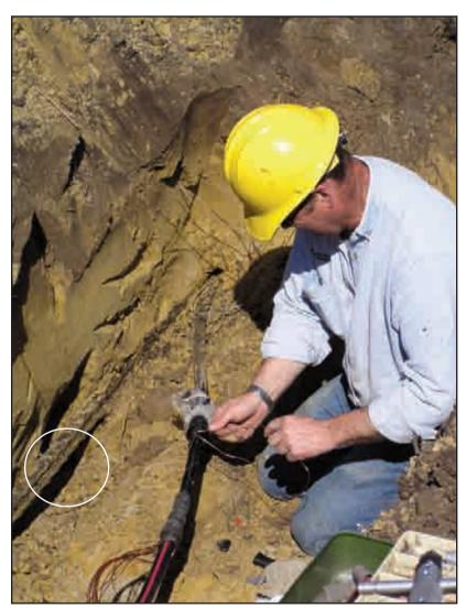
Mike Wavra, lead lineman, makes the splice from the existing underground cable to the new cable in the splice pit. The existing underground line is a three-phase line; the other two cables are also visible in the pit (marked by circle).
