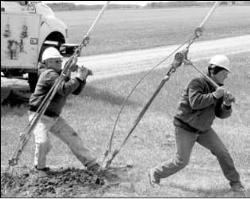
Upper Right: As the new wires are tied into place and still de-energized, everything is bonded together with grounds for protection, in case a new wire would come in contact with an existing energized wire.
