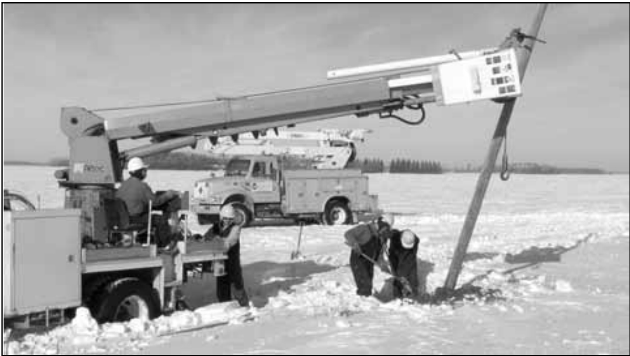
Above: A Red Lake Electric line crew work to reset the single phase poles out at an angle to make room for the new multi phase poles.
