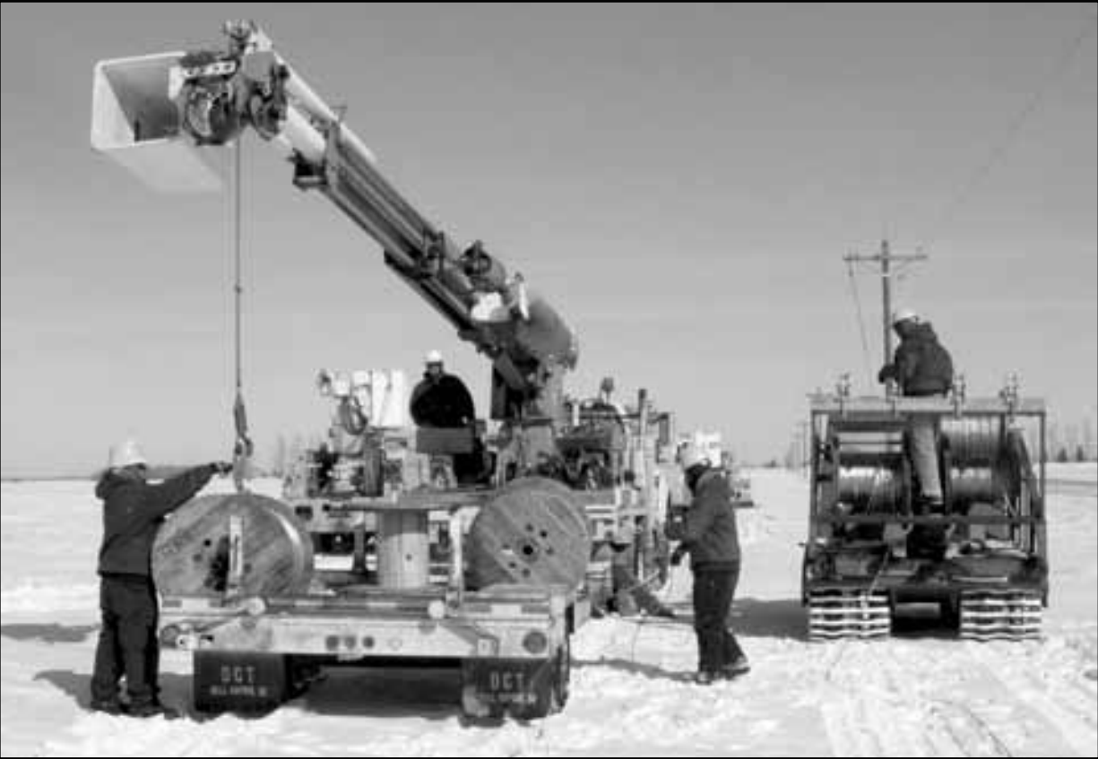
Above: A Red Lake Electric line crew work to reset the single phase poles out at an angle to make room for the new multi phase poles.
