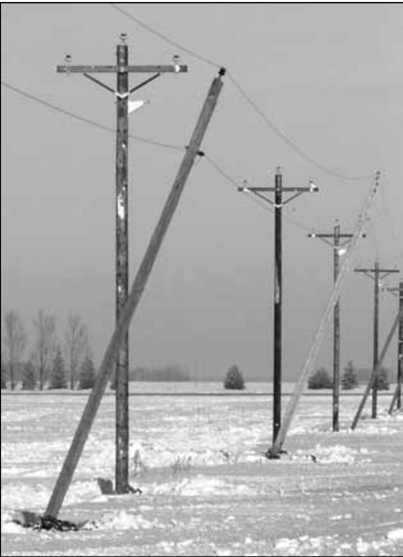
Above: A Red Lake Electric line crew work to reset the single phase poles out at an angle to make room for the new multi phase poles.
