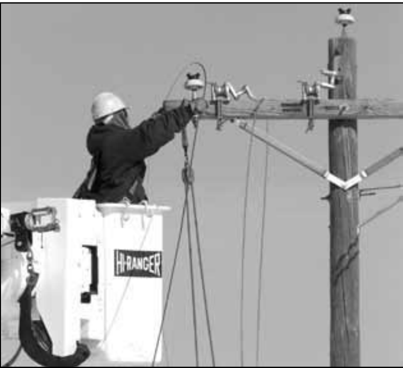
Lower Right: Troy Schmitz, lineman, sets the new wire onto a stringing block. As the wire is strung out and pulled to proper tension the stringing block rolls the wire.
