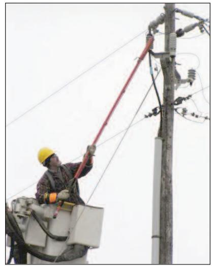
Mike Wavra uses an insulated fiberglass "shotgun" stick to disconnect the other end of the underground cable where it terminates on the riser pole.
