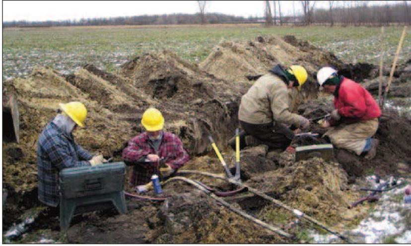
Once the cable is totally disconnected and grounded, the repair splice can be made to the wire. The linecrew works to make the splices on two cables that had faulted. Once the splices are complete the trench is filled and the line switching is restored to the normal positions and the cable can be re-energized. These cable faults occurred on a line northeast of Red Lake Falls on a Sunday afternoon affecting approximately 50 customers at the time of the fault.
