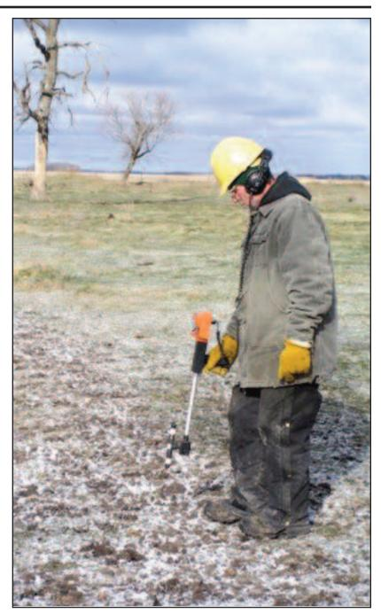
Ira Cota, lineman, uses an underground locator to determine the path of the underground wire.
