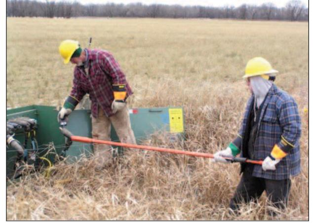
Once the underground fault location has been determined the cable needs to be exposed to splice the cable. Brett Knott, apprentice lineman (in the trench) and Roger Valley, crew foreman, work to uncover the underground cable.
