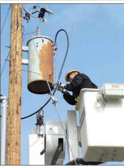
Alan Cota, lead lineman, works to connect the service wires to the transformer at the bin site. The electrical needs for aeration bins can be great in terms of amperage but short in terms of duration. Often the need only lasts for one or two months following harvest.
