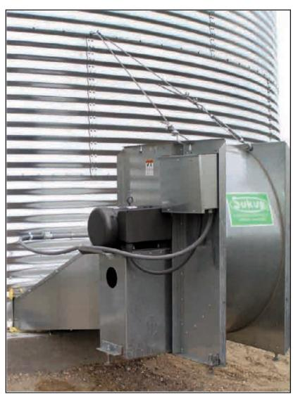
The grain bins at this site are equipped with 10 HP motors on the aeration fans. There certainly has been a need for aeration, as of late, because of the wet conditions.
