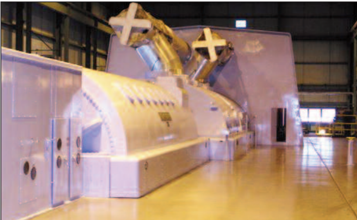
Pictured is the turbine generator of Unit II at the Milton R. Young Station. It is a Westinghouse generator with a maximum output of 455,000 kilowatts. Construction costs of Unit II, completed in 1977, was $251.7 million. Unit II consumes approximately 8,500 tons of lignite daily. Tour participants were impressed by the cleanliness of the Young Station.
