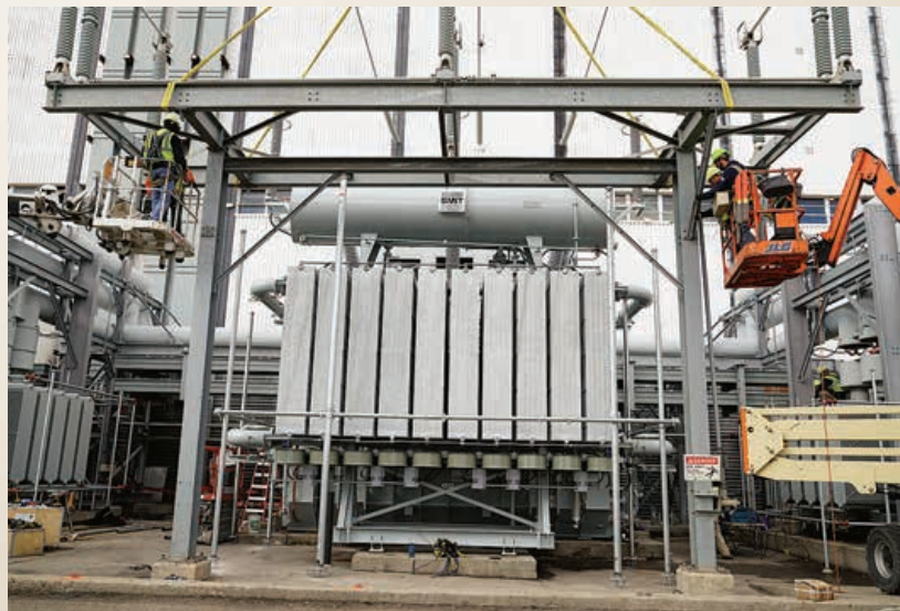
From their bucket trucks, Minnkota transmission crew members help position the new generator step-up (GSU) transformer at the Young Station.
