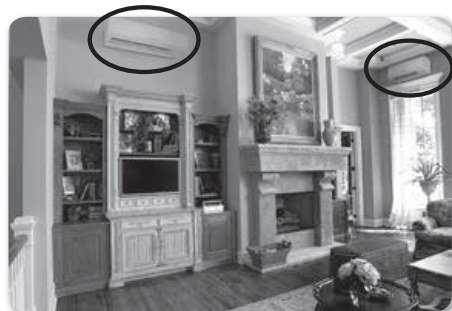
Mini-split heat pumps are popular for homes without existing ductwork. The indoor units are positioned high on the wall and come in a variety of designs to match your existing decor.
