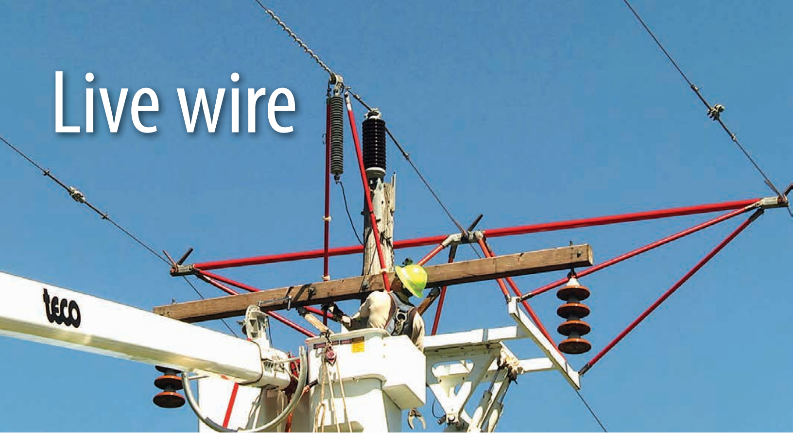
Minnkota line worker Jordan Klein works to remove an old hanging lightning arrester on an energized 69-kilovolt (kV) line.
