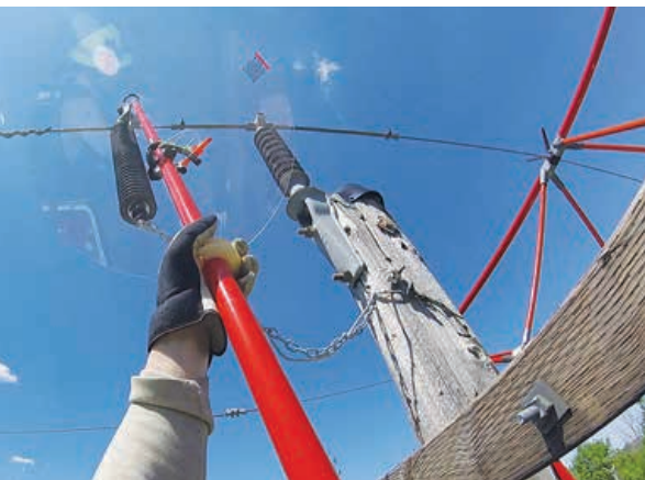
An insulated fiberglass hot stick is used to safely install blink outage mitigation equipment on energized lines.
