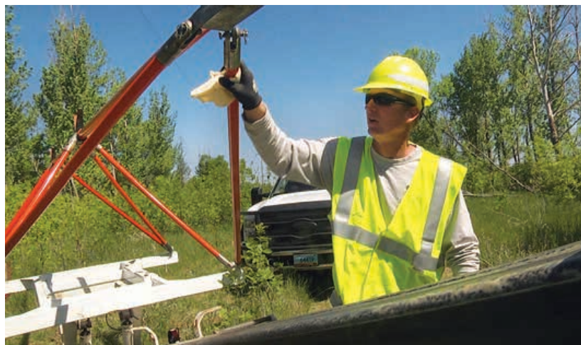
Kelly Hebl, Minnkota heavy crew foreman, cleans the insulated jib that raises the energized wires overhead so work can be completed safely.
