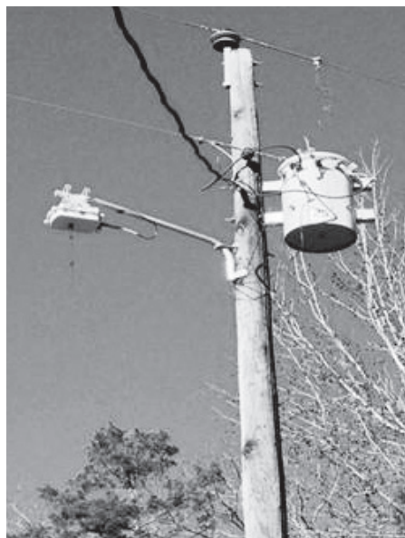
Red Lake Electric's crew will install 231 routers throughout its service territory. Routers will be installed on arms similar to what is used for mounting security lights. The routers are the communication backbone of the new AMI system.
